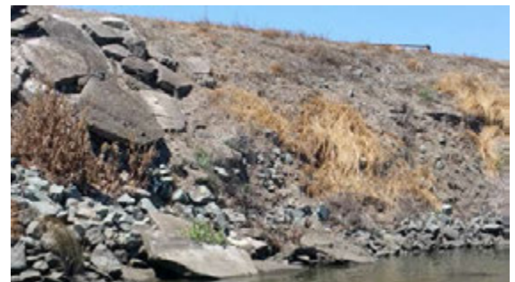
Close view of the erosion.
