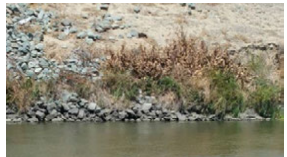
Close view of the erosion. Note river rocks and vegetation at the levee toe.
