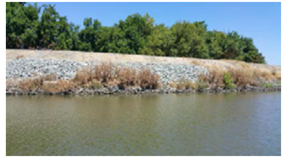
View of the repaired site. Note the new erosion at the levee toe.
