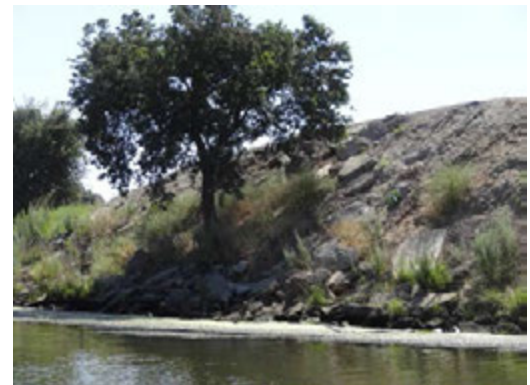
Front view of the site. Note existing broken concrete on the upper slope as well as on the lower slope and at the toe.
