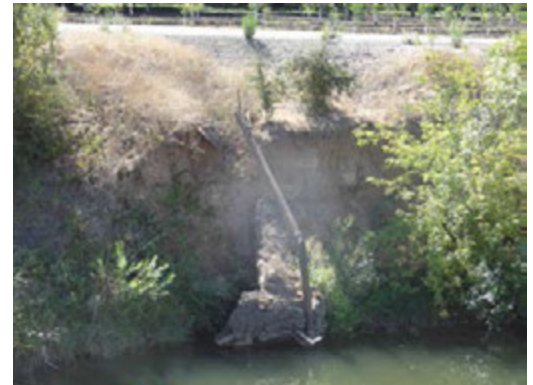
Close view of the erosion. Note the drainage pipe at the site.
