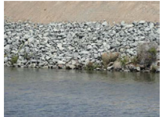
Front view of the repaired erosion site.
