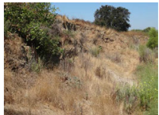
Close view of the erosion. Levee crest is approximately 8 feet above the erosion.
