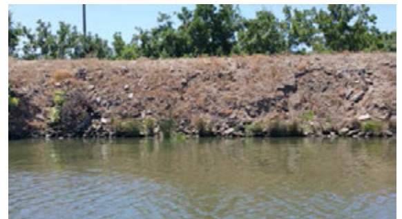
Close view of the erosion.
