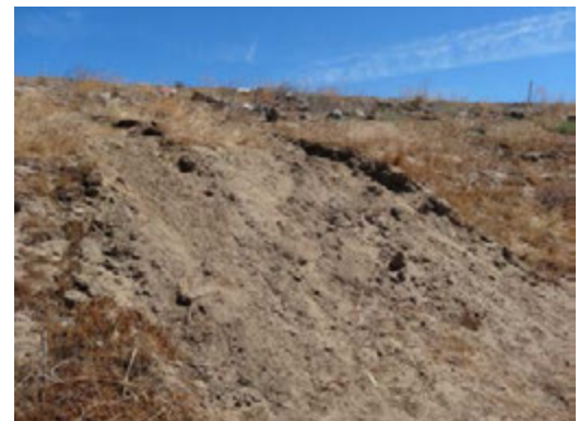
Direct view of the levee slope. Note the loose soil possibly caused by runoff.
