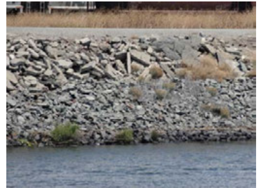
Close view of the repaired erosion site.
