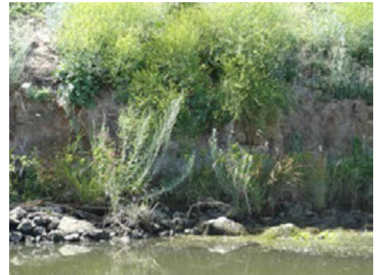
Close view of the pocket erosion.
