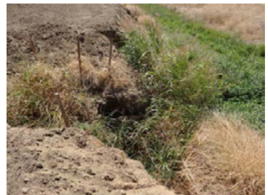
The erosion site has been repaired but a minor erosion at the lower bank slope is still visible.
