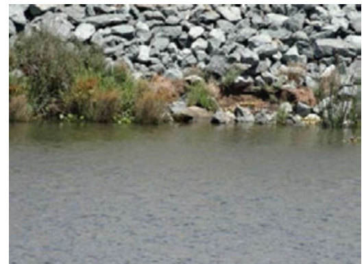
Close view of the repaired erosion site. Note the minor erosion at the water edge.
