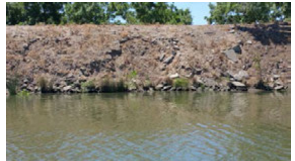
Close view of the erosion.
