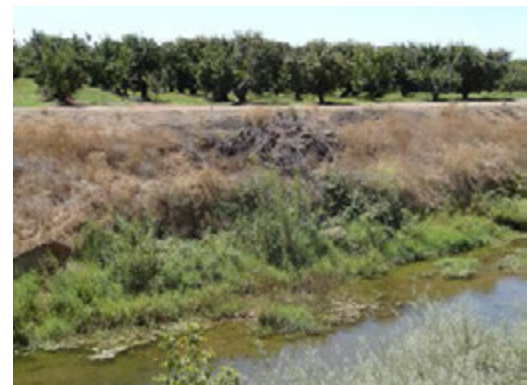
Close view of the erosion.
