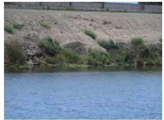
Front view of the erosion site. Note the vegetation at the levee toe and on the lower slope.
