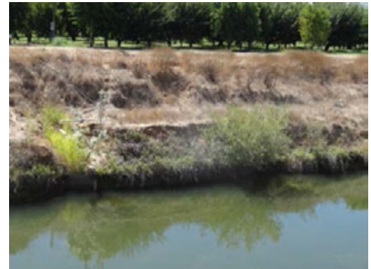
Front view of the erosion at the berm.
