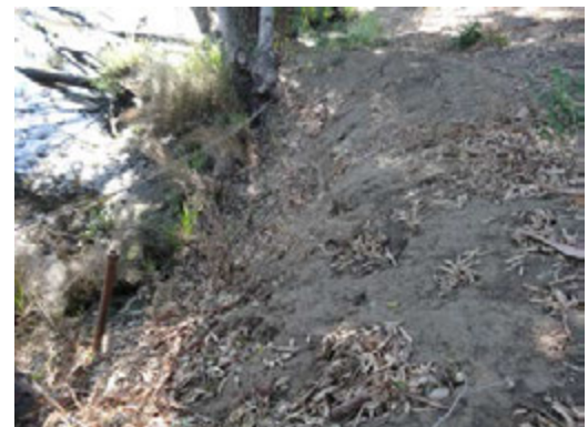
Close view of the erosion at the levee toe.
