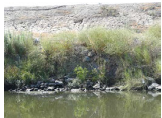
Close view of the erosion.
