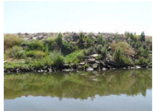
Front view of the site. Previously placed rip rap slipped, exposing the underlying soils and creating a pocket.
