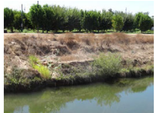
Closer view of the erosion.
