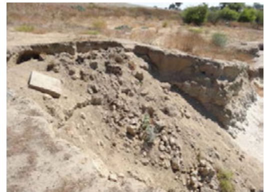
Close view of the pocket erosion.
