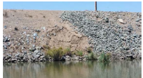
Close view of the erosion.
