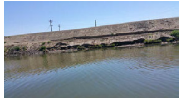
Front view of the erosion.
