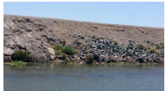
Close view of the erosion. The upstream end of the site is protected by riprap revetment.
