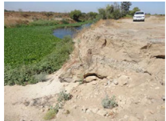
Looking upstream. Note the pocket erosion.
