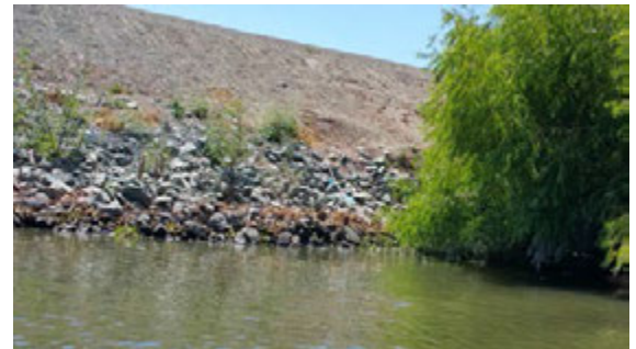
Close view of the repaired erosion site.
