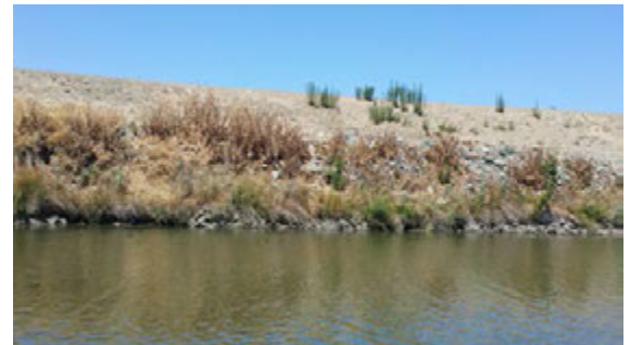
Close view of the erosion.
