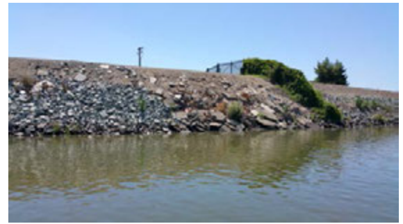
Front view of the erosion site. Note the concrete blocks and vegetation.
