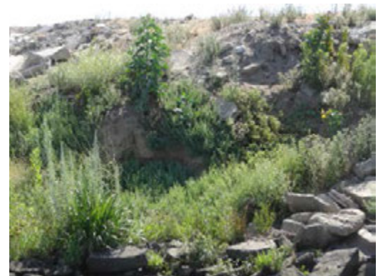
Front view of the site. Rip rap no longer adequately protecting levee slope.
