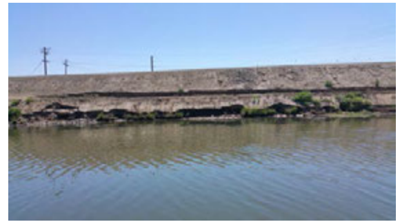
Front view of the erosion site. Note the new cut at the middle levee slope.
