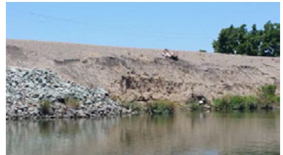
Front view of the erosion.
