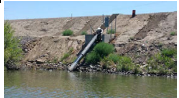
Close view of the repaired erosion site.
