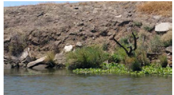
Close view of the pocket erosion.
