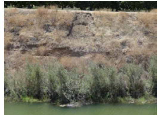
Close view of the erosion.
