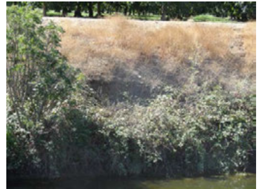
Front view of the pocket erosion.
