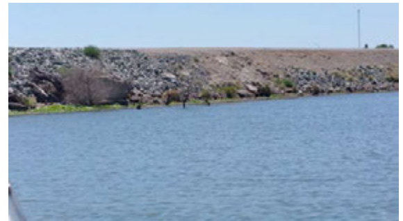
Close view of the erosion. Note the protection on the lower levee slope.
