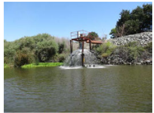
Front view of the site. The irrigation pipe is functioning and leaking water at the site.
