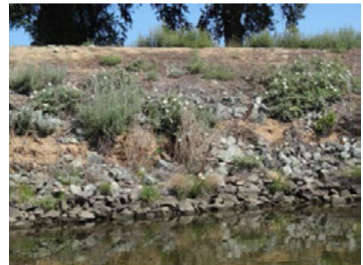
Close view of the erosion.
