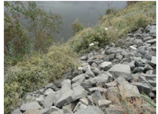
The erosion is not visible from the levee top. The levee slope is protected by riprap rocks.
