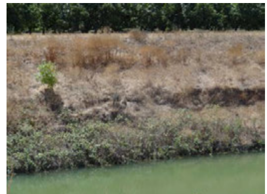
Front view of the erosion.
