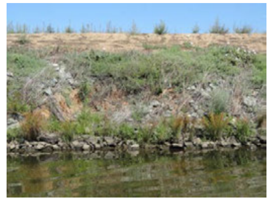
Front view of pocket erosion. Note the vegetation and riprap at the site.
