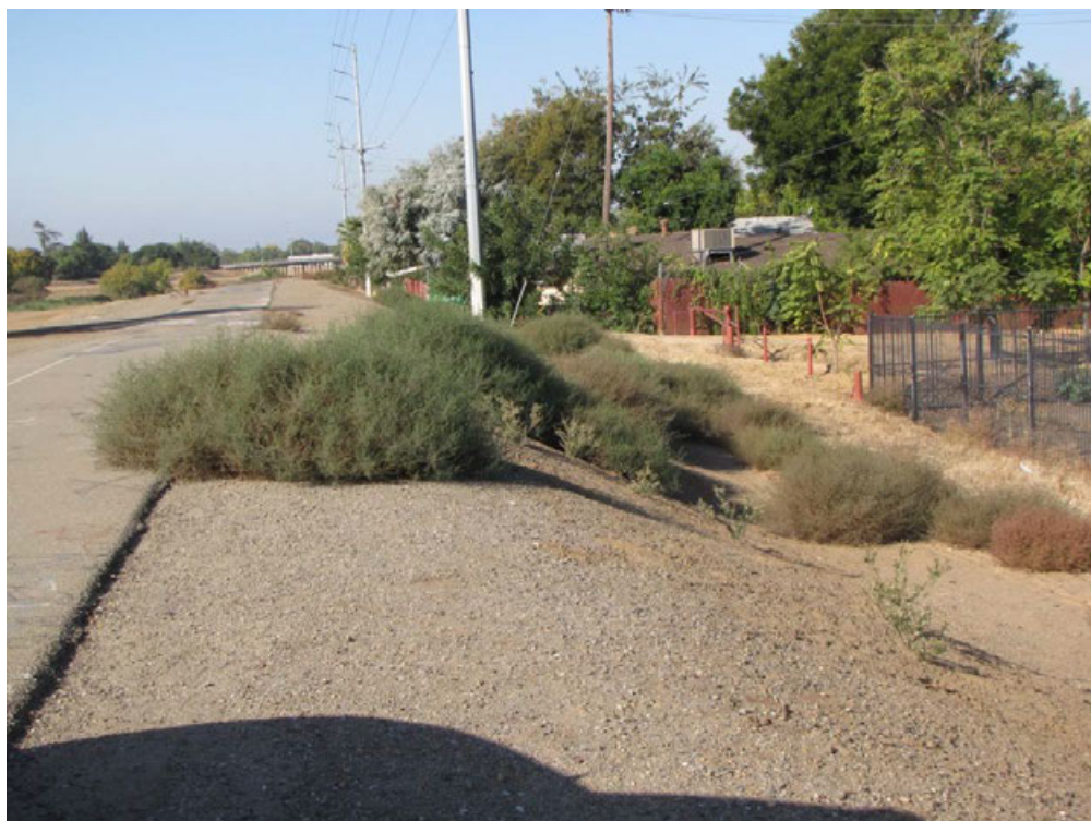
Minimally Acceptable Maintenance: Grass or brush partially obstruct visibility and access
