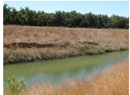
Close view of the erosion.
