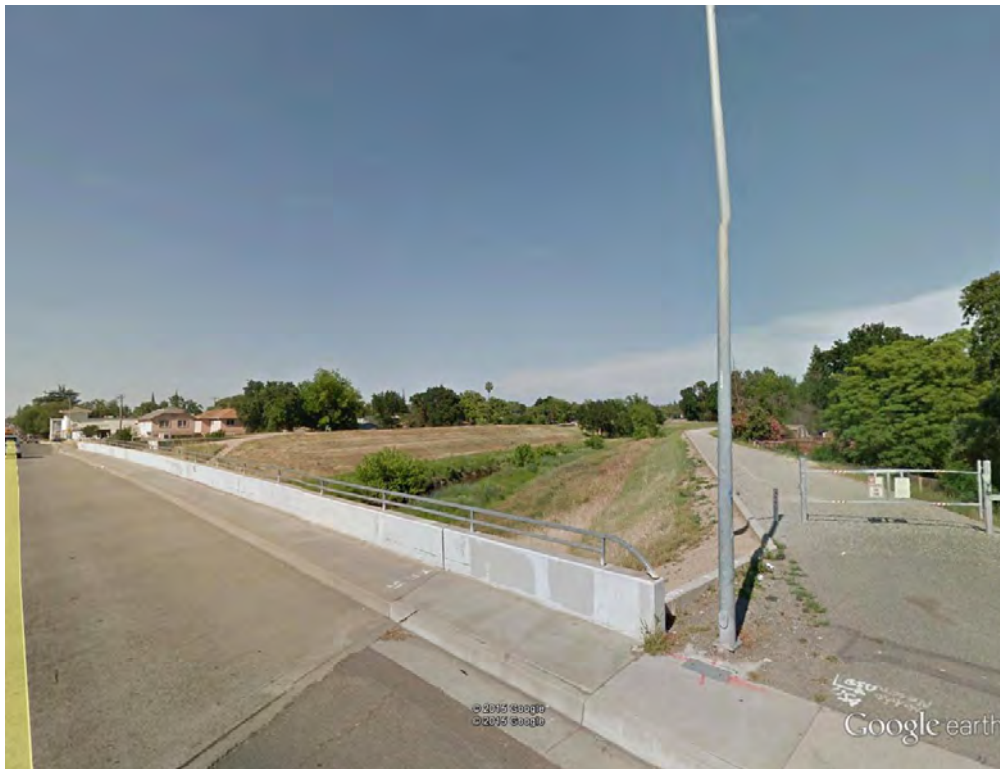
Site Photo 2- View of Arcade Creek Channel and North and South Levee. View is to the northeast (upstream) from Rio Linda Boulevard.
