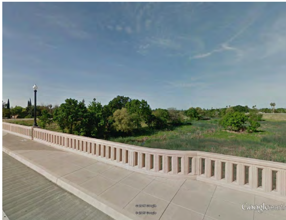
Site Photo 4- View of Arcade Creek Channel and North and South Levee. View is to the west (downstream) from Norwood Avenue.
