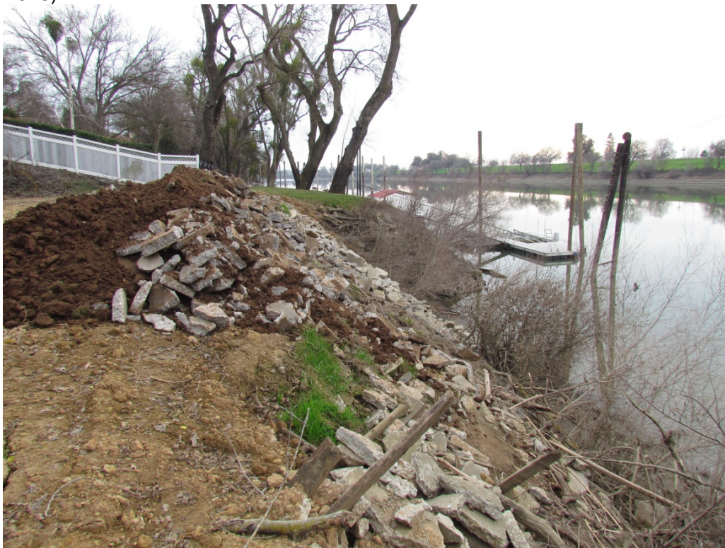
Photo 2: Soil and demolished concrete placed on the waterside levee berm and river bank (DWR Inspection – January 28, 2015)
