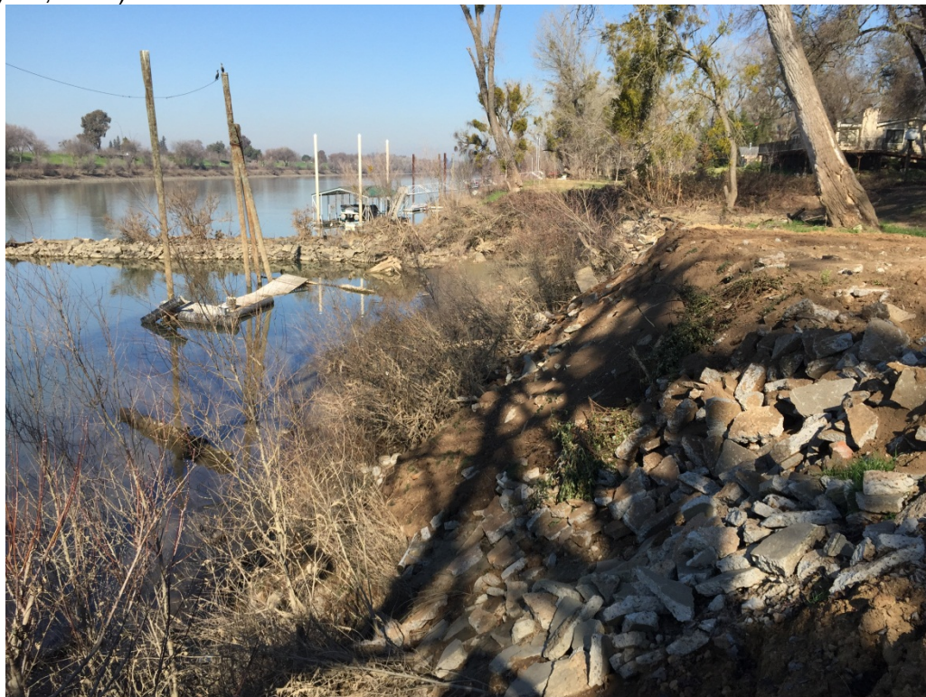
Photo 3: Soil and demolished concrete placed on the waterside levee berm and river bank (CVFPB site visit – January 30, 2015)
