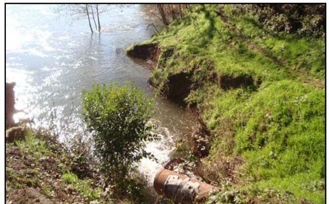
Photo 8) This photo shows a high flow event that occurred in December 2010, during which the stage of the American River was 10 to 12 inches below the culverted drainage. Note that the high river flows have eroded the banks around culvert. Photo taken 12/16/2010.
