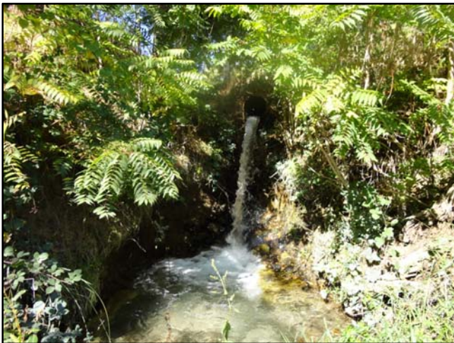
Photo 6) This view is of the outflow of the unnamed drainage where it emerges from the culvert and drops eight to ten feet into an eroded scour pool flanked by invasive plant species. Step ponds will be placed to within two to three feet of the outflow and invasive vegetation will be removed and replaced with native plant species. Photo taken 10/1/2014.
