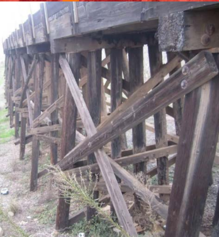
Existing Bend in Railroad
