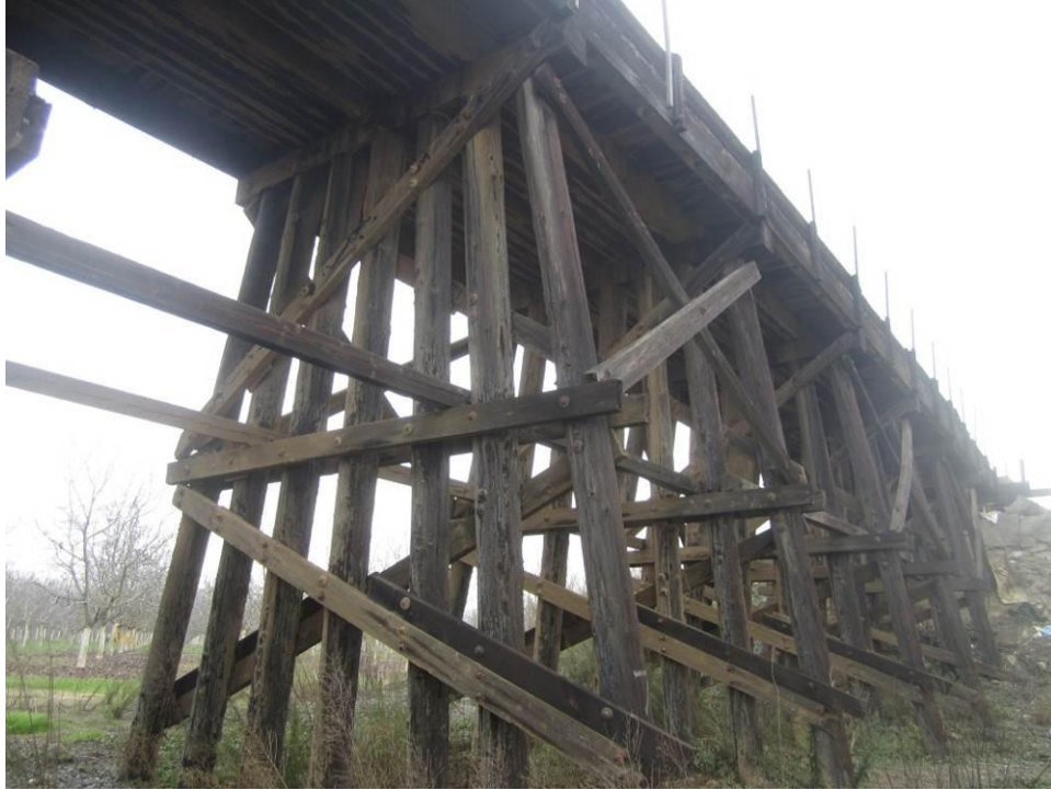
PHOTO 31: View at of typical bent, looking TT South.
