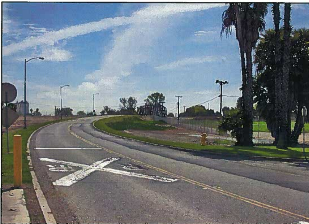
VP3. Looking southeast from Navy Drive/Washington Street intersection at the Navy Drive Bridge.
