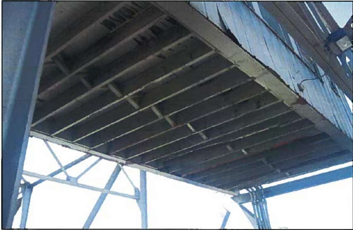
Bridge Control House
