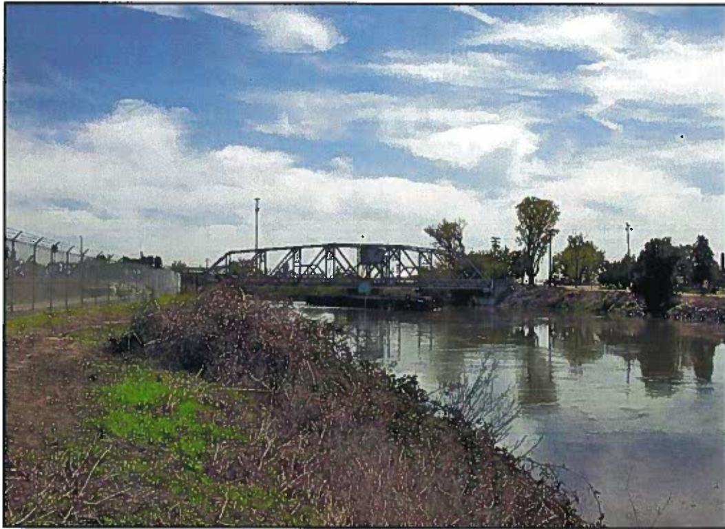
VP1. From riverbank looking northeast at Navy Drive Bridge.
