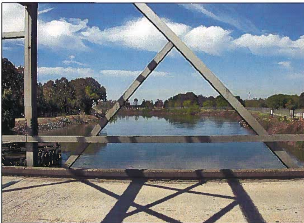
VP5. From Navy Drive Bridge looking southwest.
