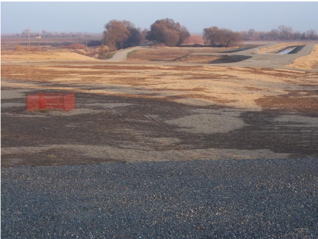
Photograph 4: Looking east from top of adjacent levee to beginning of Elkhorn Canal. The temporary transition structure to be removed is in the foreground and fenced with orange fence.
