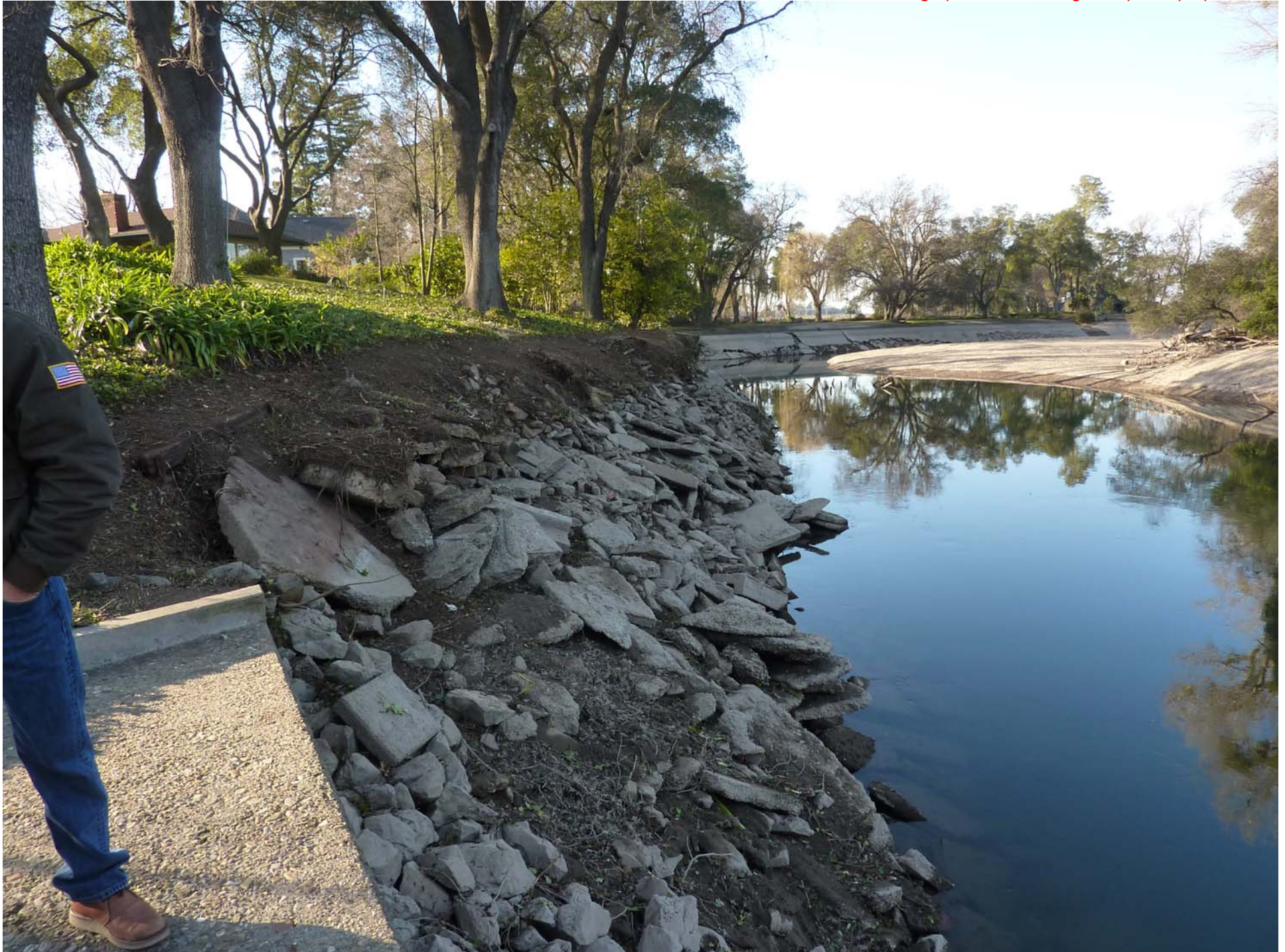
Attachment C - Photograph of the Existing Slumped Riprap
