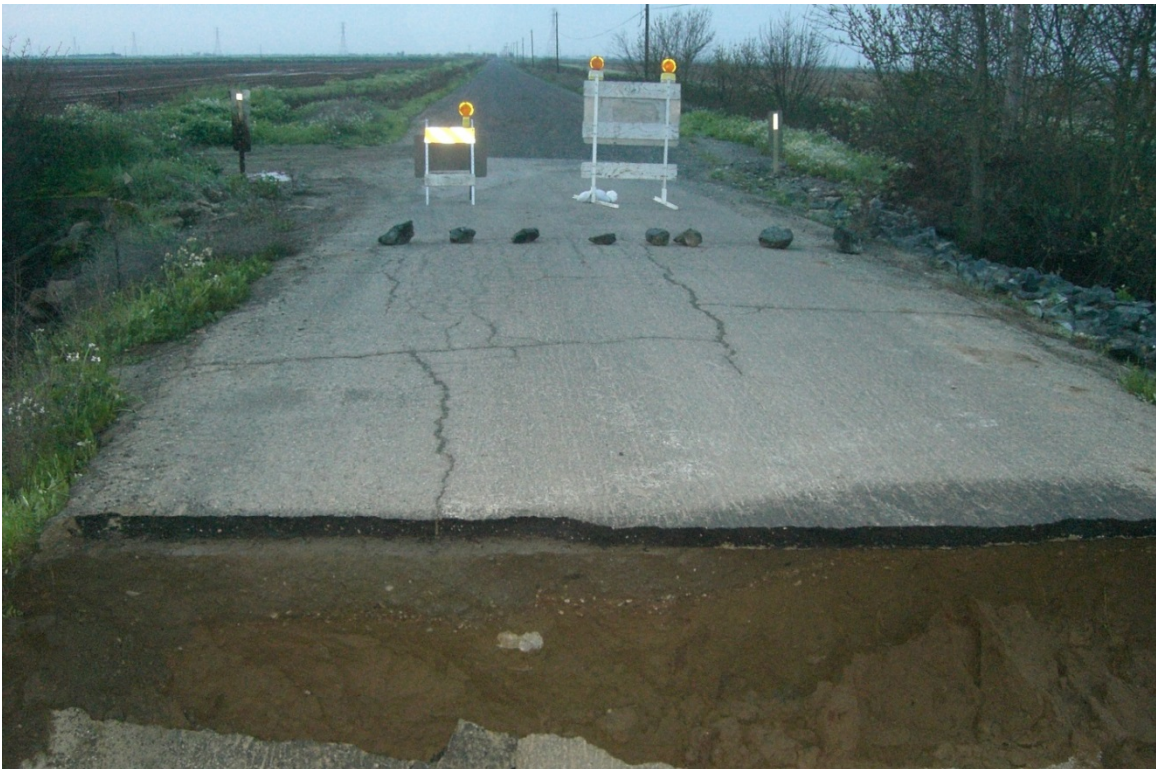
Photo 9: Brewer Rd – Western Pipe Collapse – March 2010
