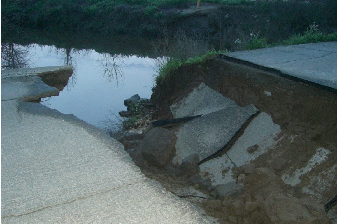
Photo 10: Brewer Rd – Western Pipe Collapse – March 2010
