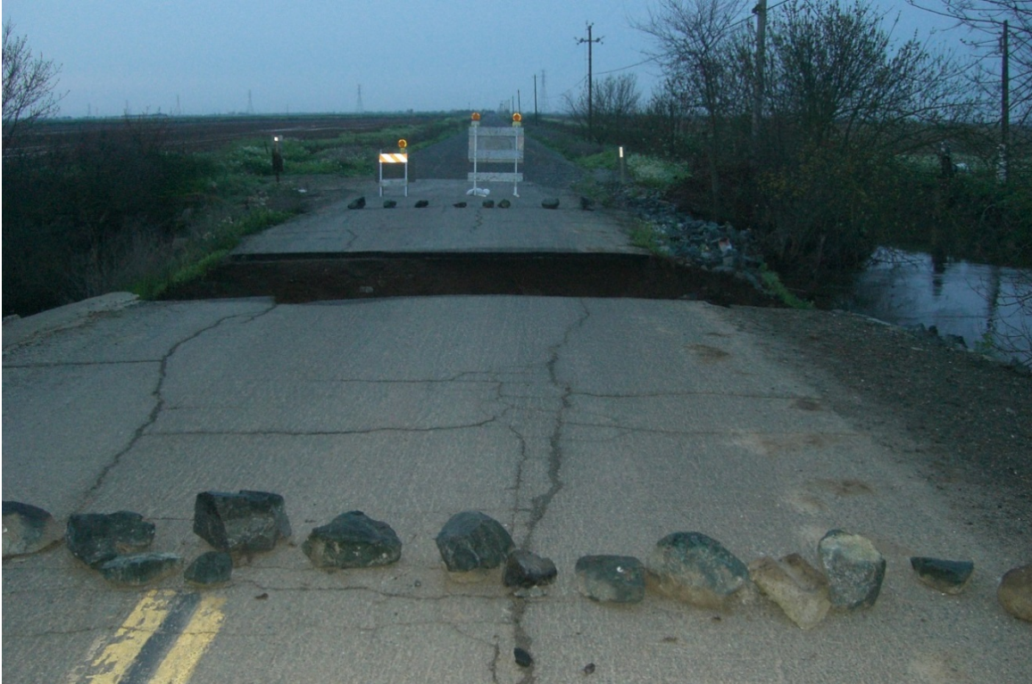
Photo 8: Brewer Rd – Western Pipe Collapse – March 2010
