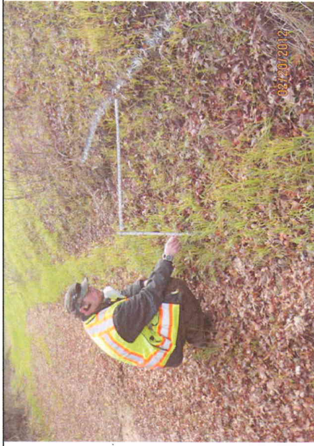
Inspect ID: NIC2_2012_p_0183 Title: USACE_CESPK_NIC2_2012_p_0183_1.jpg Rated Item: 3. Encroachments Caption: Waterside toe cut, 24 inches tall, 100 feet long.- Likely due to maintenance vehicles. (U)
