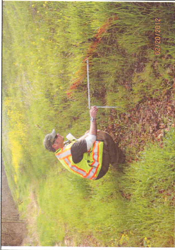
Inspect ID: NIC2_2012_p_0194 Title: USACE_CESPK_NIC2_2012_p_0194_1.jpg Rated Item: 3. Encroachments Caption: Start point. Waterside toe cut, up to 24 inches tall. Likely due to maintenance vehicles. End point is 196. (U)
