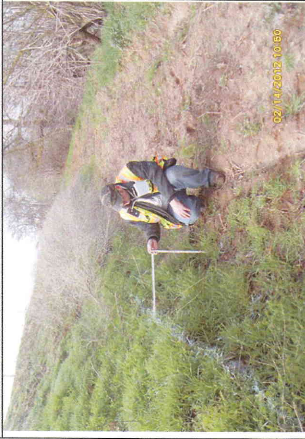
Inspect ID: NICU_2012_p_0188 Title: USACE_CESPK_NICU_2012_p_0188_1.jpg Rated Item: 3. Encroachments Caption: Waterside toe cut, 24 inches deep, 150 feet long. Likely due to maintenance vehicles. (U)
