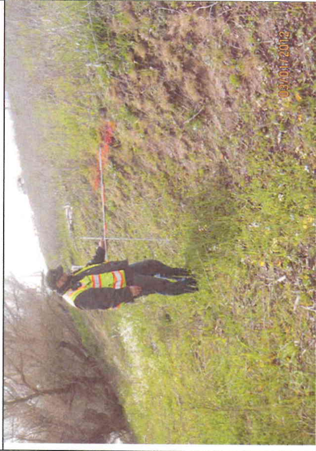
Inspect ID: NIC5_2012_p_0128 Title: USACE_CESPK_NIC5_2012_p_0128_3.jpg Rated Item: 3. Encroachments Caption: 3 foot tall waterside toe cut for 100 feet. Likely due to maintenance vehicles. (U)
