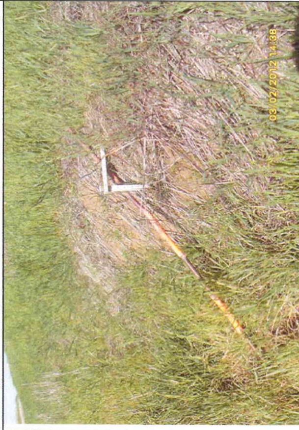
Inspect ID: NIC6_2012_p_0107 Title: USACE_CESPK_NIC6_2012_p_0107_1.jpg Rated Item: 3. Encroachments Caption: Toe cut on landside. 18 to 24 inches tall with 1:1 slope over 100 feet. (U)
