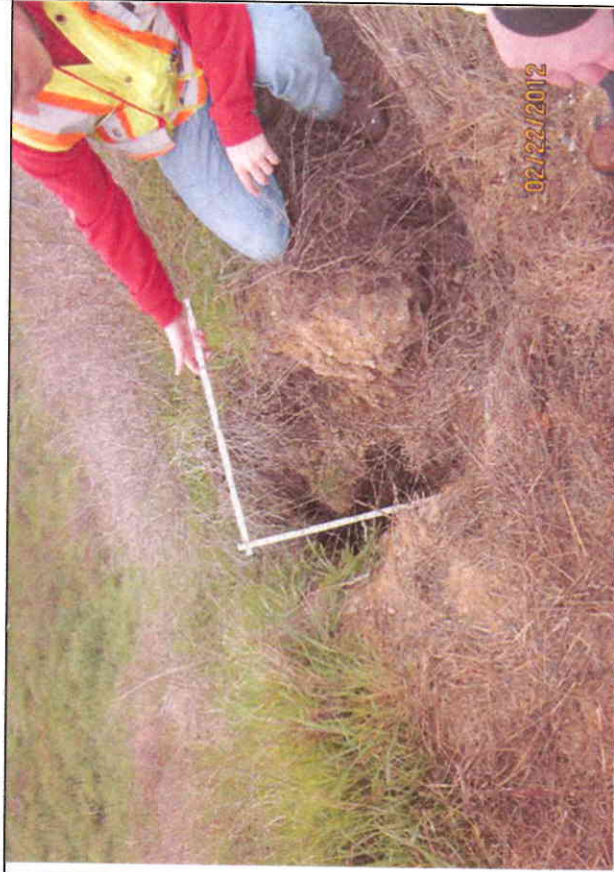
Inspect ID: NIC3_2012_p_0029 Title: USACE_CESPK_NIC3_2012_p_0029_1.jpg Rated Item: 2. Sod Cover Caption: Erosion rill on landside embankment from hinge to midslope. 24 inches wide and 30 inches deep. (U)
