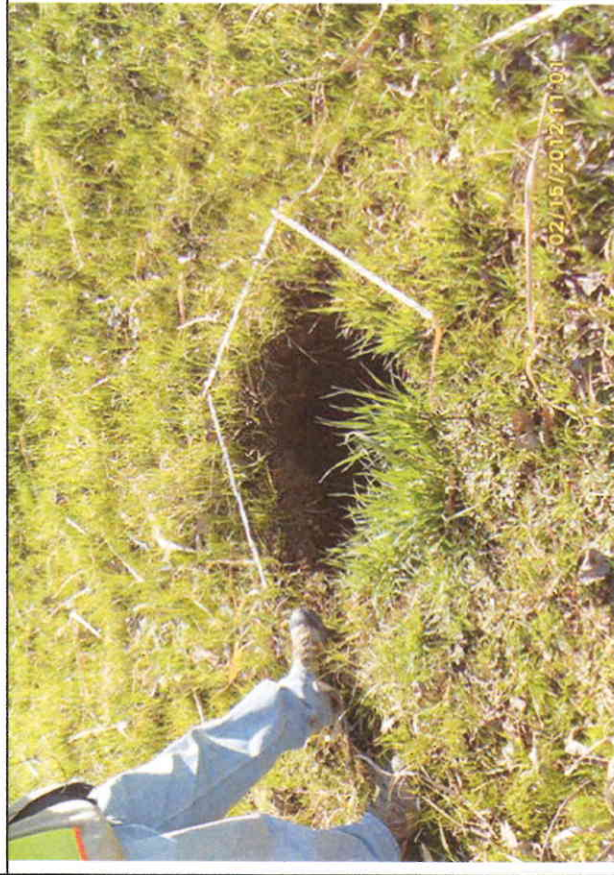
Inspect ID: NICU_2012_p_0375 Title: USACE_CESPK_NICU_2012_p_0375_1.jpg Rated Item: 8. Depressions/ Rutting Caption: Hole at waterside toe, 3 feet diameter, 3 feet deep. (U)
