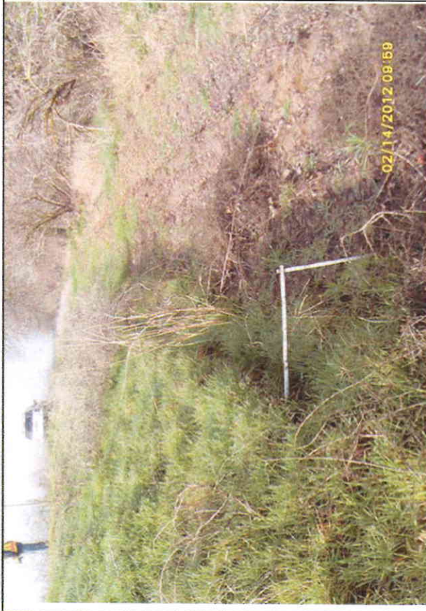
Inspect ID: NICU_2012_p_0165 Title: USACE_CESPK_NICU_2012_p_0165_1.jpg Rated Item: 3. Encroachments Caption: Waterside toe cut, 2 feet deep, 200 feet long. Likely due to maintenance vehicles. (U)
