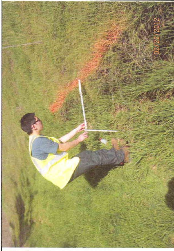
Inspect ID: NIC3_2012_p_0150 Title: USACE_CESPK_NIC3_2012_p_0150_1.jpg Rated Item: 3. Encroachments Caption: Waterside toe cut, 12 to 24 inches tall. Likely due to maintenance vehicles. (U)
