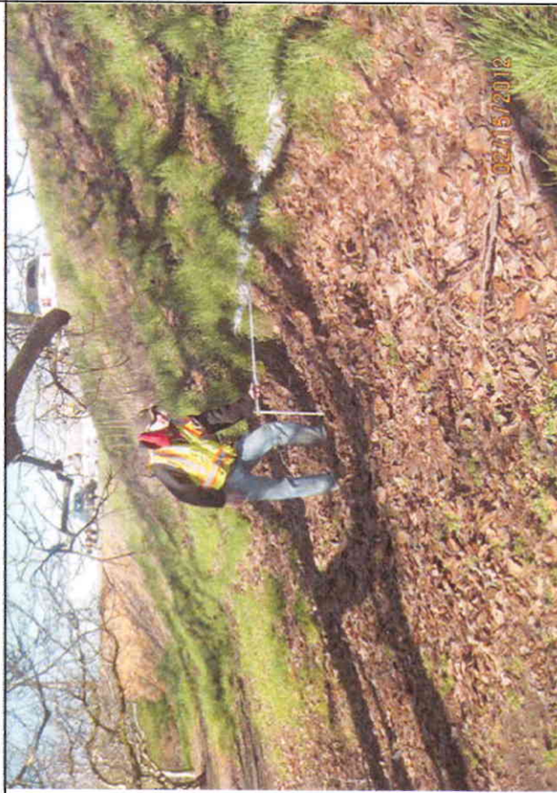
Inspect ID: NICU_2012_p_0347 Title: USACE_CESPK_NICU_2012_p_0347_1.jpg Rated Item: 3. Encroachments Caption: Landside toe cut, 24 inches deep, about 100 to 150 feet long. (U)
