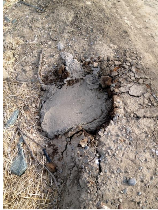
Representative view of cement slurry used to backfill hole resulting from pole relocation.
