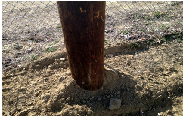
Detail of backfilled soil surrounding relocated pole.
