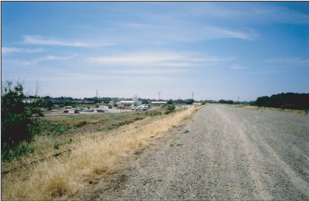
Photo 2-6. Reach E, looking downstream from eastern end of reach. Note concrete processing batch plant on landside of the levee at left, as well as railroad tracks evident in vegetation on levee slope.
