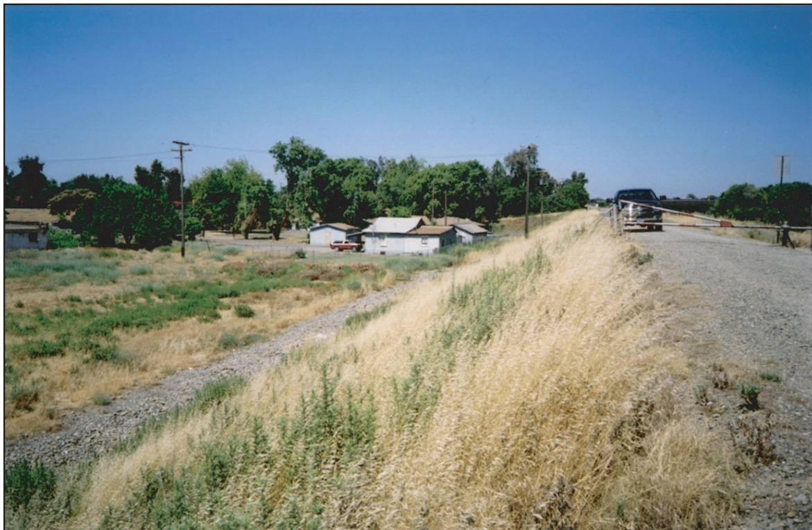
Photo 2-3. Reach C, looking downstream (west) at western end of reach toward Reach B. Note rental residences and rock toe trench on landside of levee (at left).
