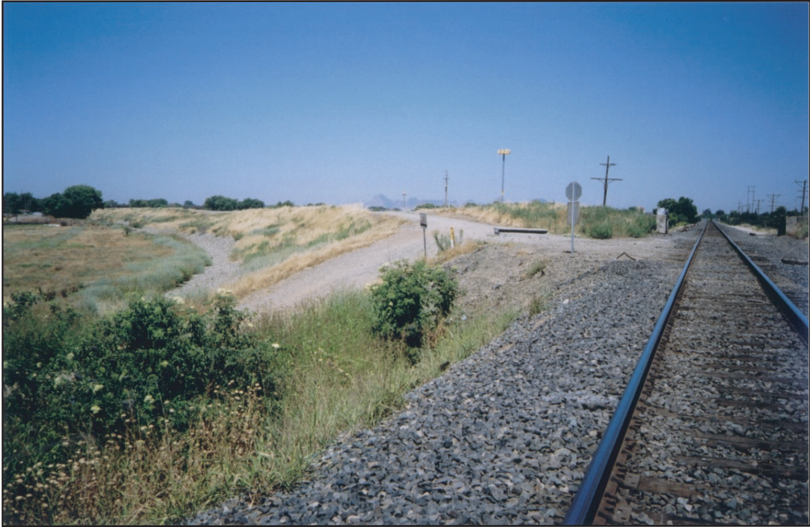
Photo 2-5. Reach D, looking downstream (west) from the railroad (old SPRR). The levee and track intersect at the floodgate headwalls at right. Note the rock toe trench at the base of the levee. Also note elderberry shrubs in the foreground and Sutter Buttes in the background.
