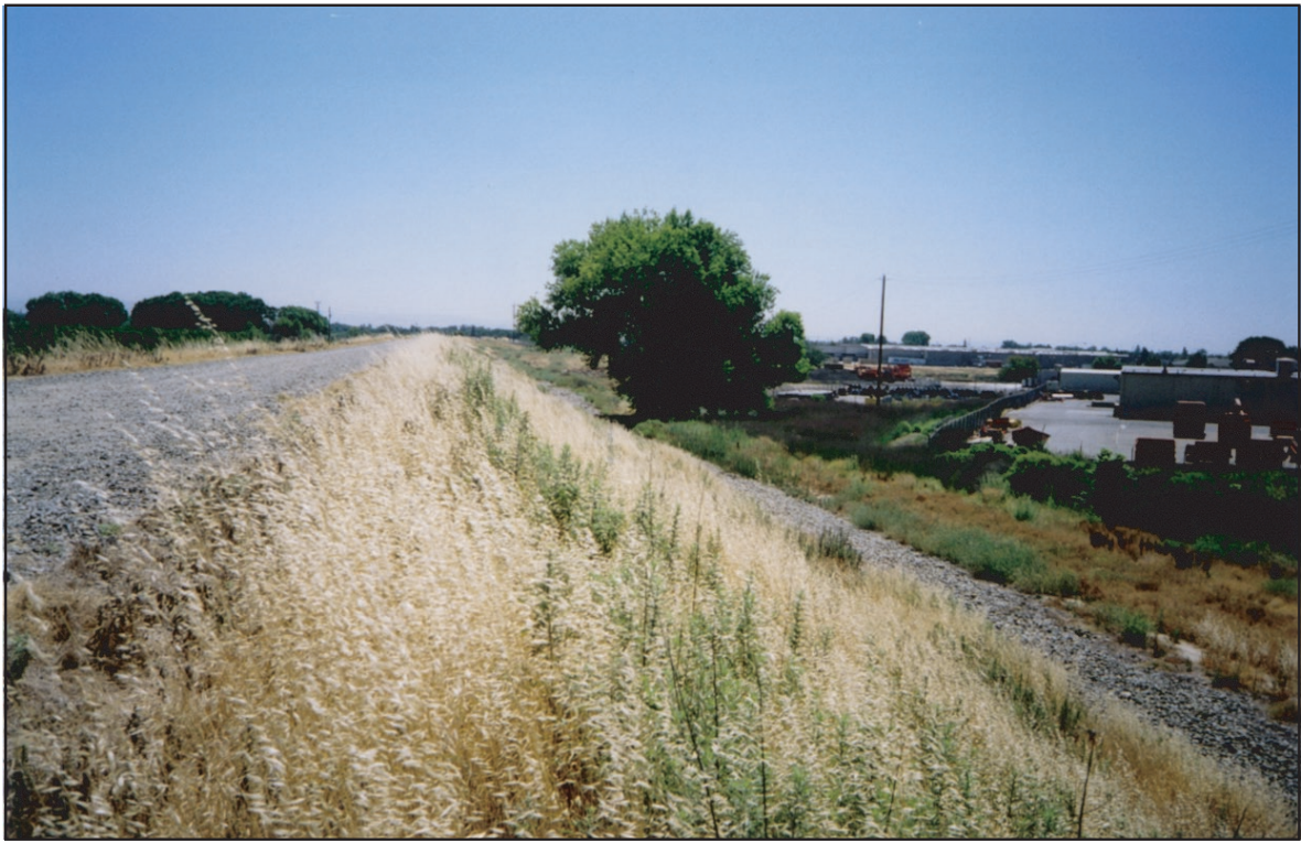
Photo 2-4. Reach C, looking upstream (east) near western end of reach. Note Caltrans yard, vegetation, and rock toe trench on landside of the levee.
