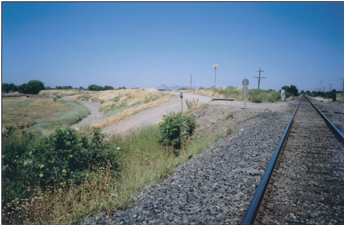
Photo 2-5. Reach D, looking downstream (west) from the railroad (old SPRR). The levee and track intersect at the floodgate headwalls at right. Note the rock toe trench at the base of the levee. Also note elderberry shrubs in the foreground and Sutter Buttes in the background.
