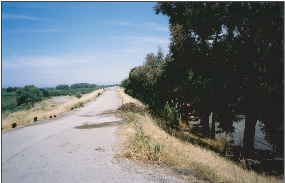
Photo 2-2. Reach B, looking upstream east with mobile home park on landside of levee. Note treeline at levee toe.
