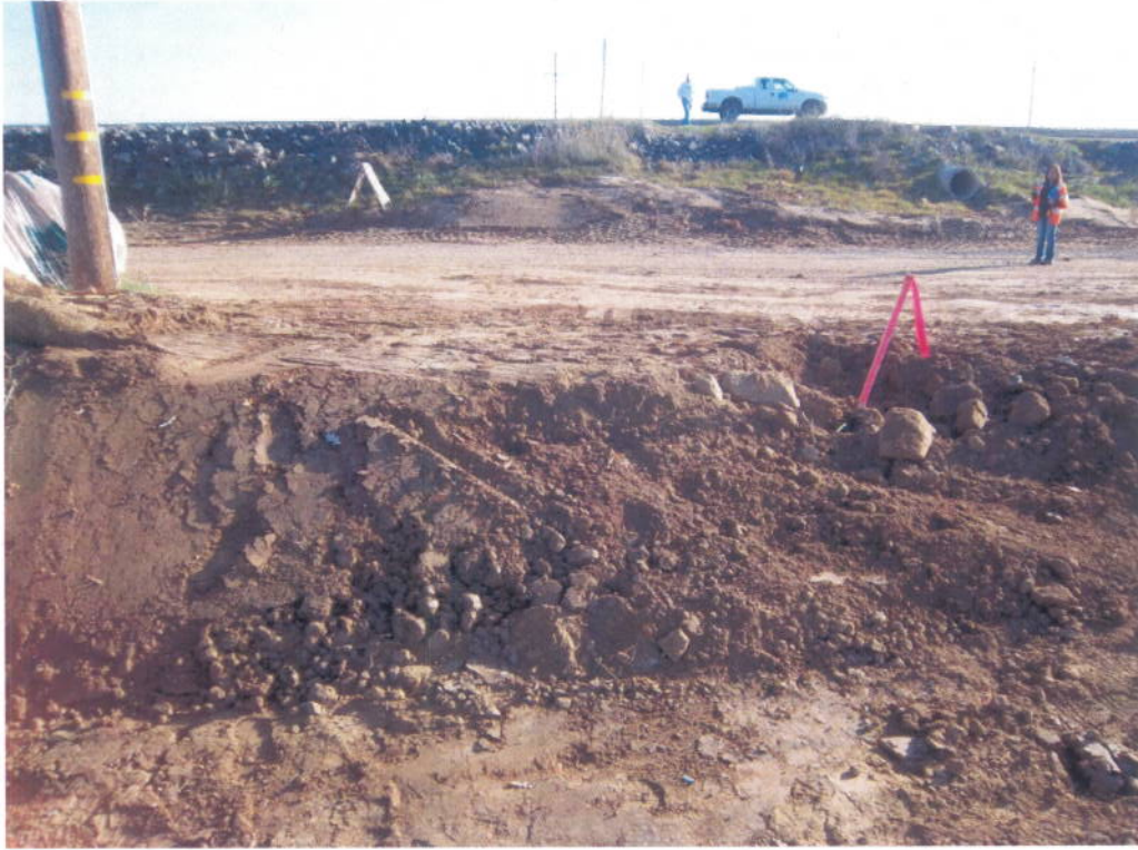
Photograph 3: Looking east toward Garden Highway from Lauppe South River Pump.
