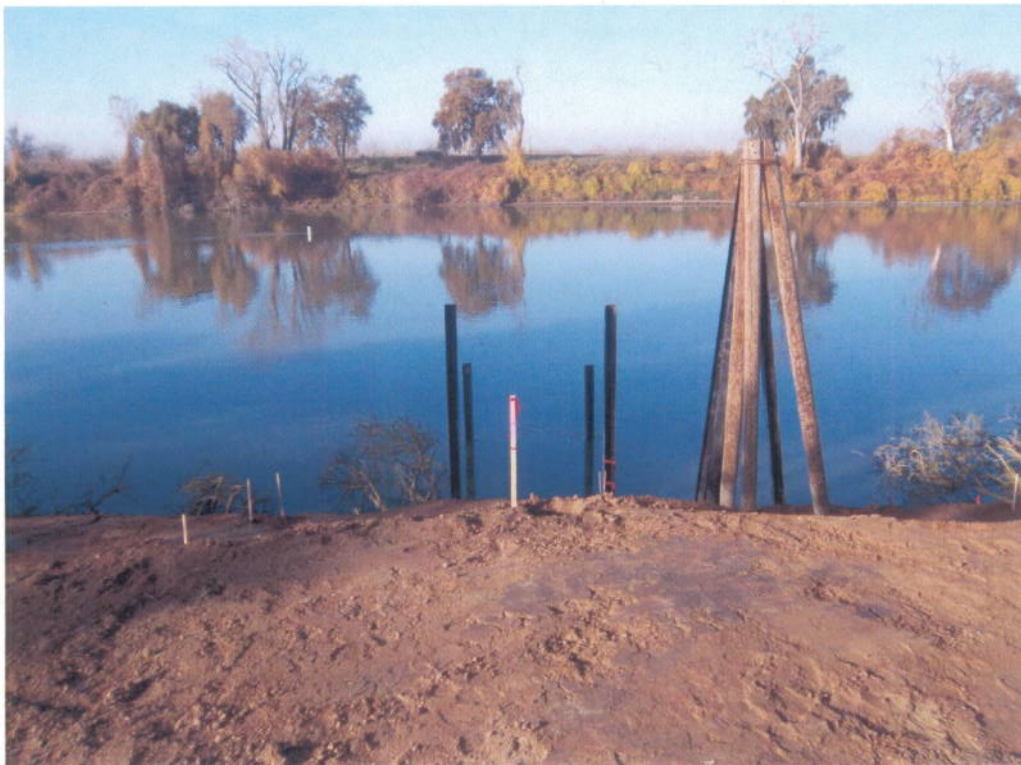
Photograph 2: Looking west at the existing piles for the Lauppe South River Pump.
