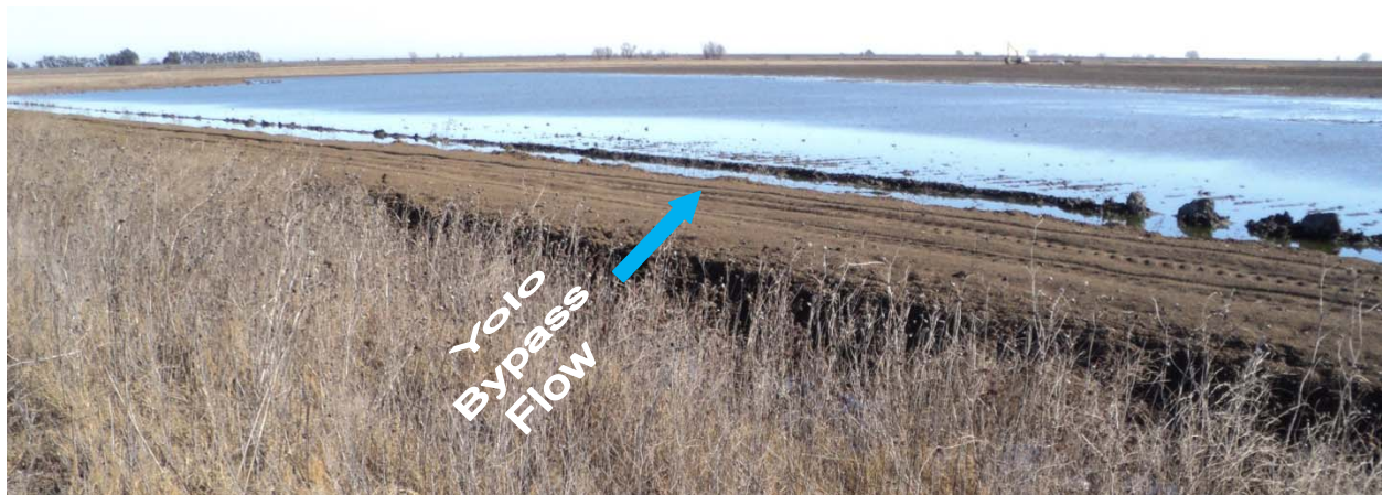
Figure 5 – Soil Berms Blocking Free Flow of Drainage (Source: Board staff site visit 2.2.2012)
