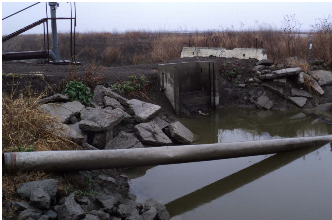
Figure 7 – Drainage Structure Blocking Free Flow of Water (Source: Board staff site visit 1.20.2012)
