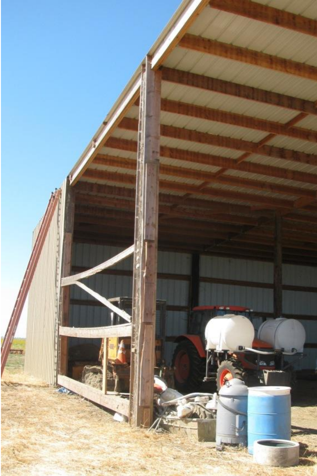
Damaged side of barn, panels blown off by wind
