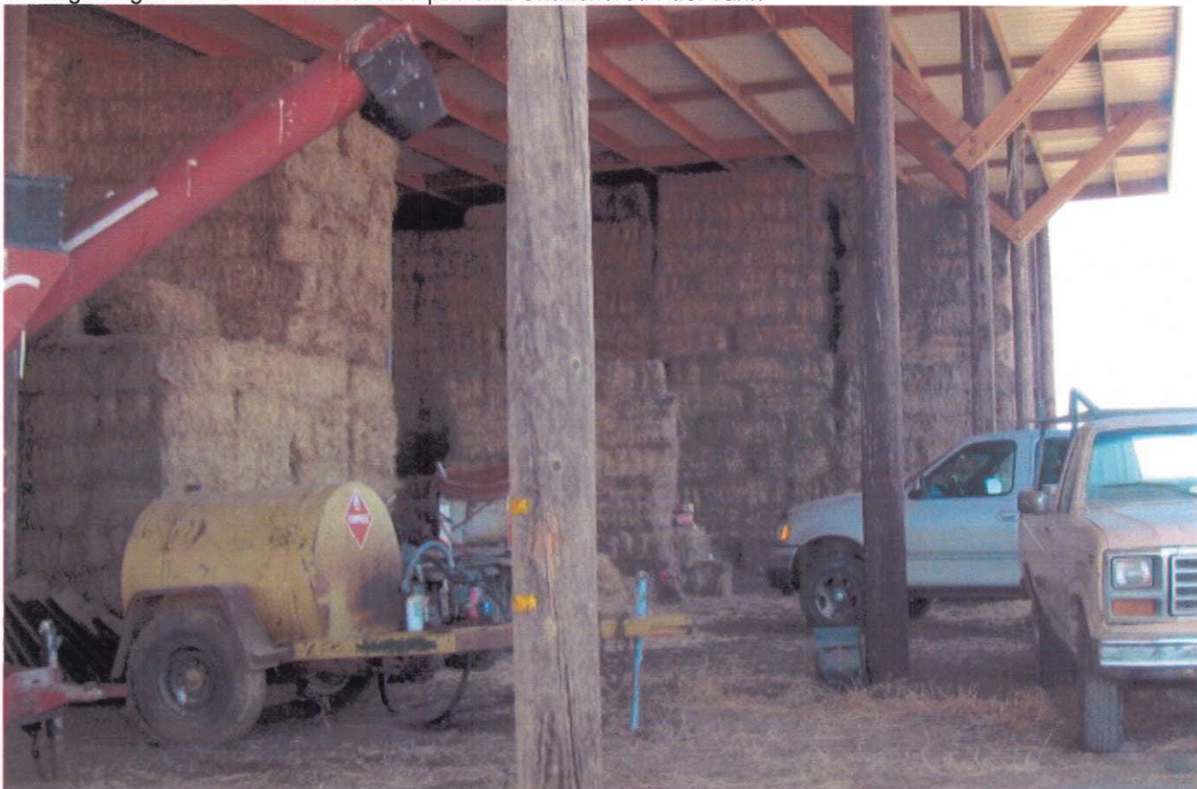
Damaged Agricultural Barn on elevated pad and Unanchored Fuel Tank
