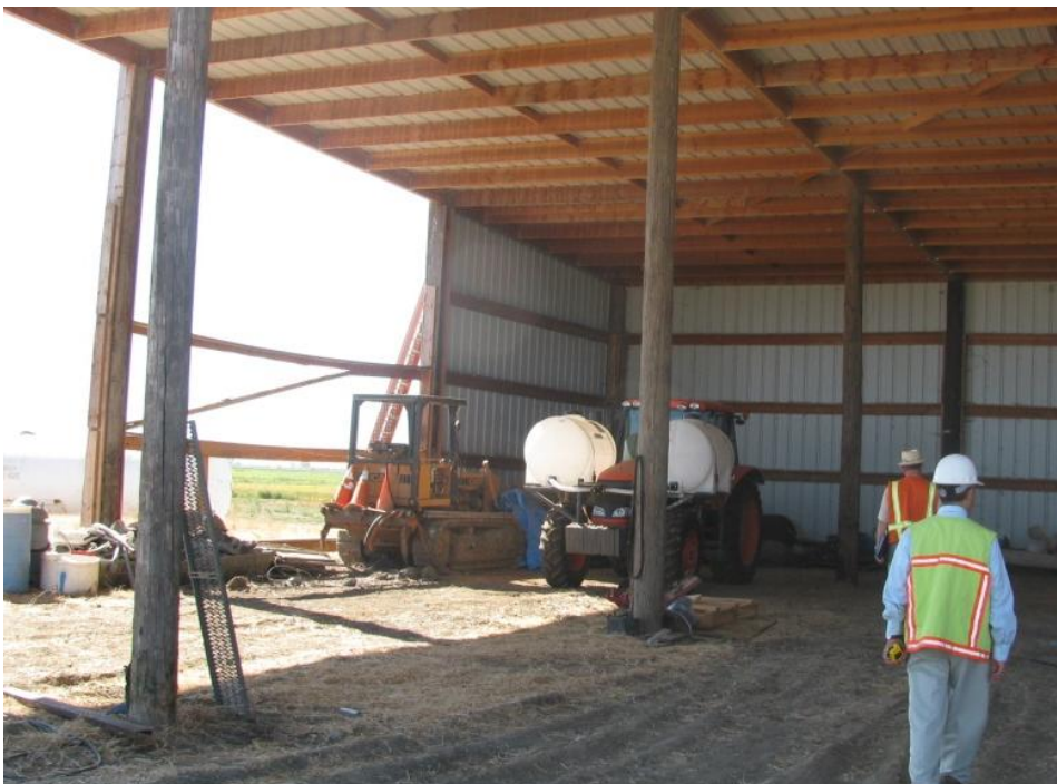
Damaged side of barn, panels blown off by wind
