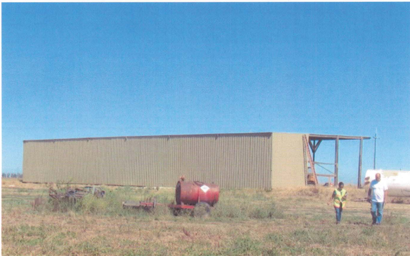
Damaged Agricultural Barn on elevated pad and Unanchored Fuel Tank
