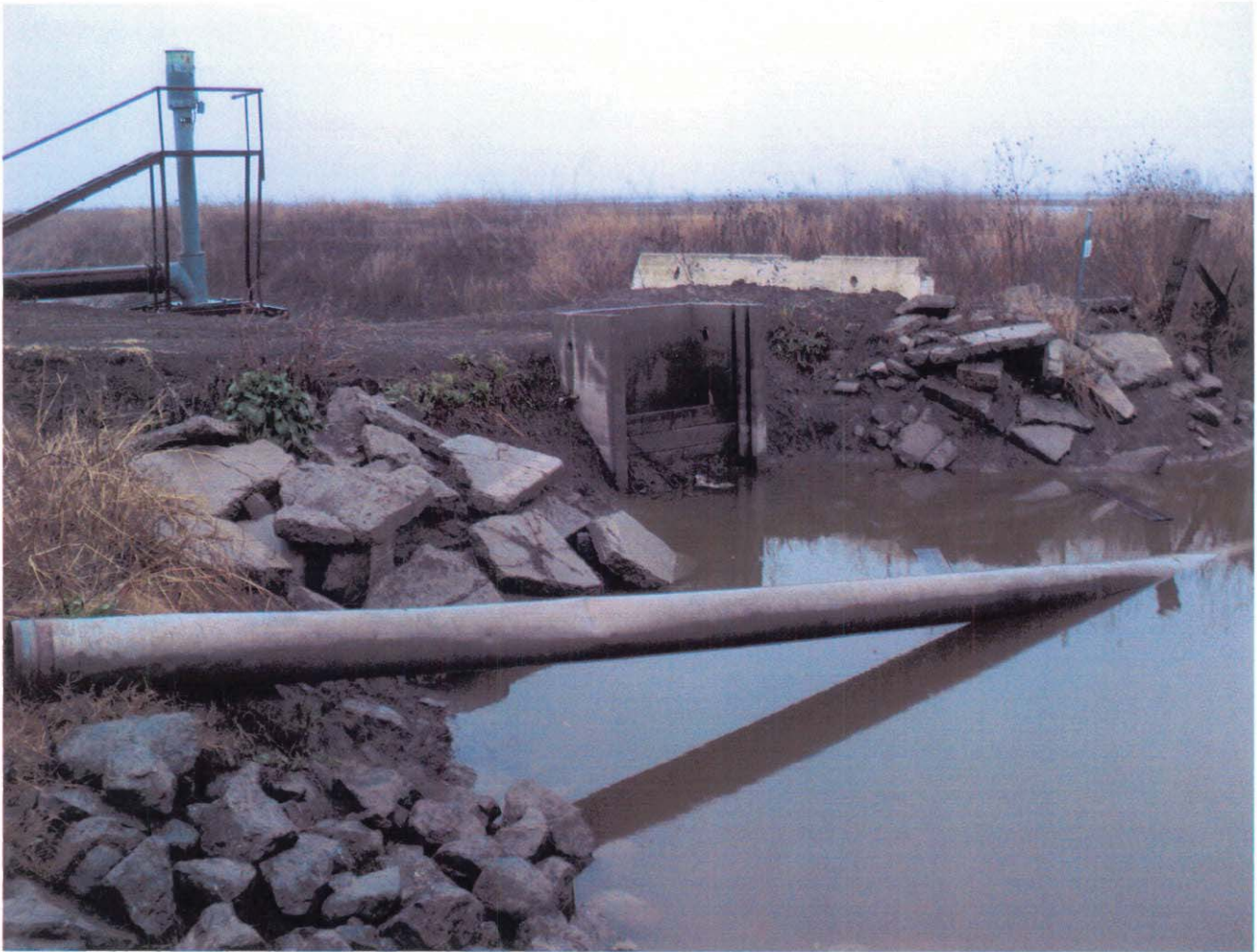
Drainage structure blocking free flow of water.
