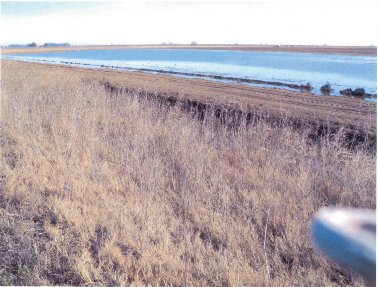
Soil Berm Blocking Drainage
