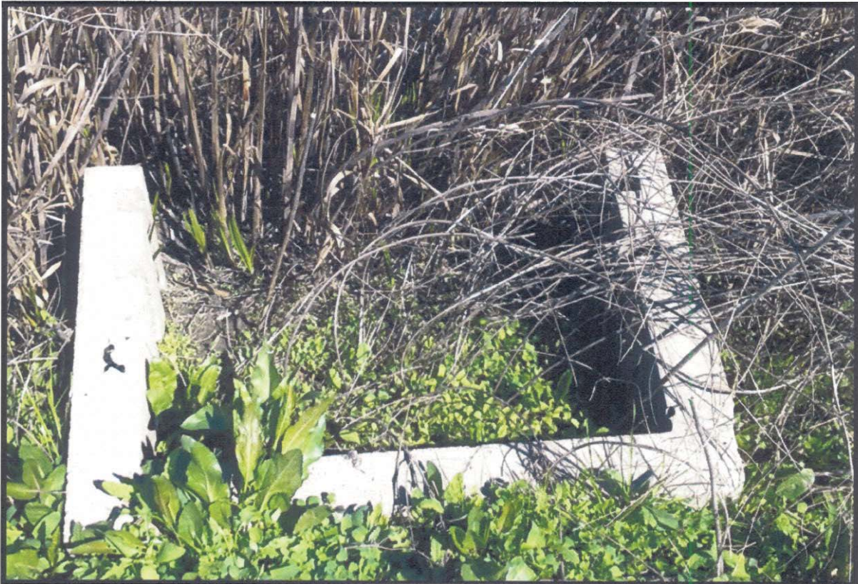
Un-maintained picture of drainage box on northern property Picture taken on 3/23/12
