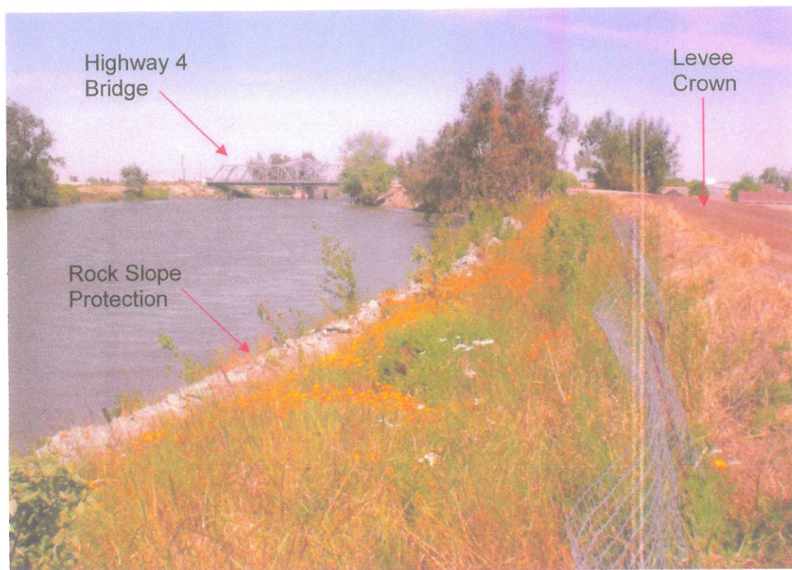
Photograph 2 - View downstream from SJR RM 42.3R, depicting typical water-side erosion repair.
