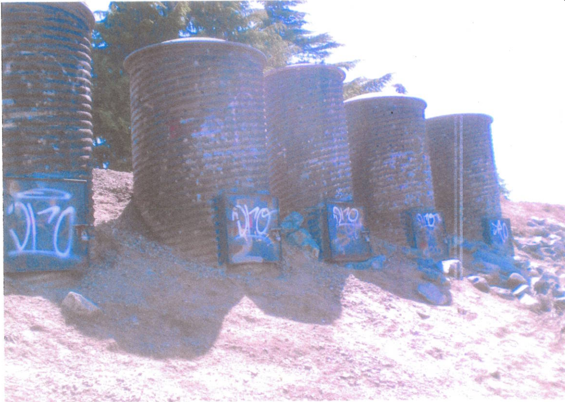
Photograph 9 – View southward on waterside levee slope at SJR RM 42.3R, showing storm drain outlet structure siphon breakers.
