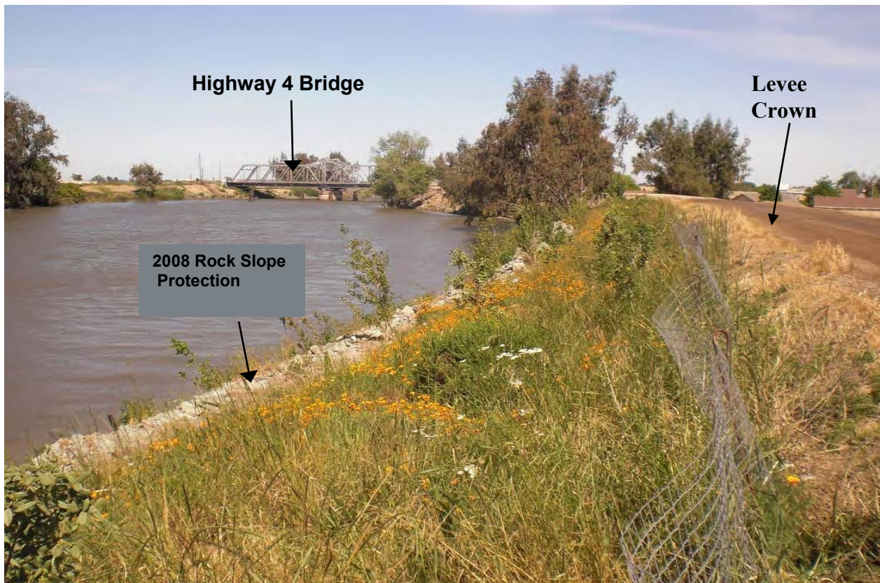
Figure 10. View of Erosion Repair at RM 42.3R Completed in 2008 and Located Along Approximately 480 feet of the 1,200 Foot Levee Repair Length.
