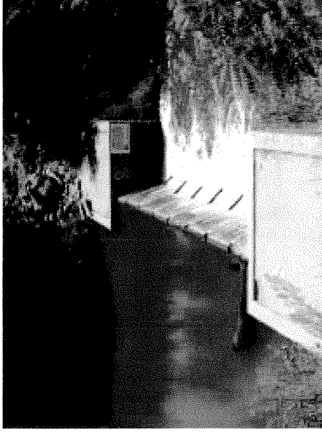
Photo D-56. Flashboards in place at Bonomo Flashboard Dam
