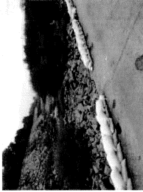
Photo D-35. View upstream across Hosie Low-flow Road Sandbags installed to provide temporary fish passage improvement.
