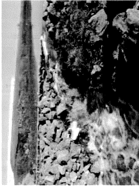
Photo D-19. At-grade view of riprap cascade downstream from Budiselich Dam
