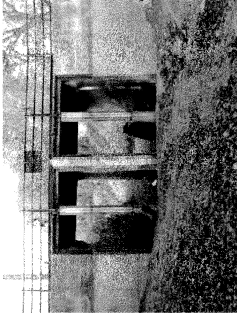
Photo D-118. Upstream view of Pezzi Flashboard Dam. Note sediment accumulation at inlet
