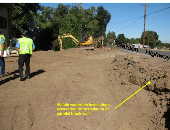
Figure 2c- Cut on waterside levee slope in preparation for block wall. Board staff site visit on September 21, 2010.
