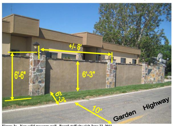
Figure 3a - New solid masonry wall. Board staff site visit June 22, 2011
