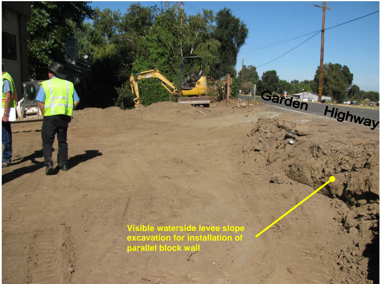
Figure 2c- Cut on waterside levee slope in preparation for block wall. Board staff site visit on September 21, 2010.
