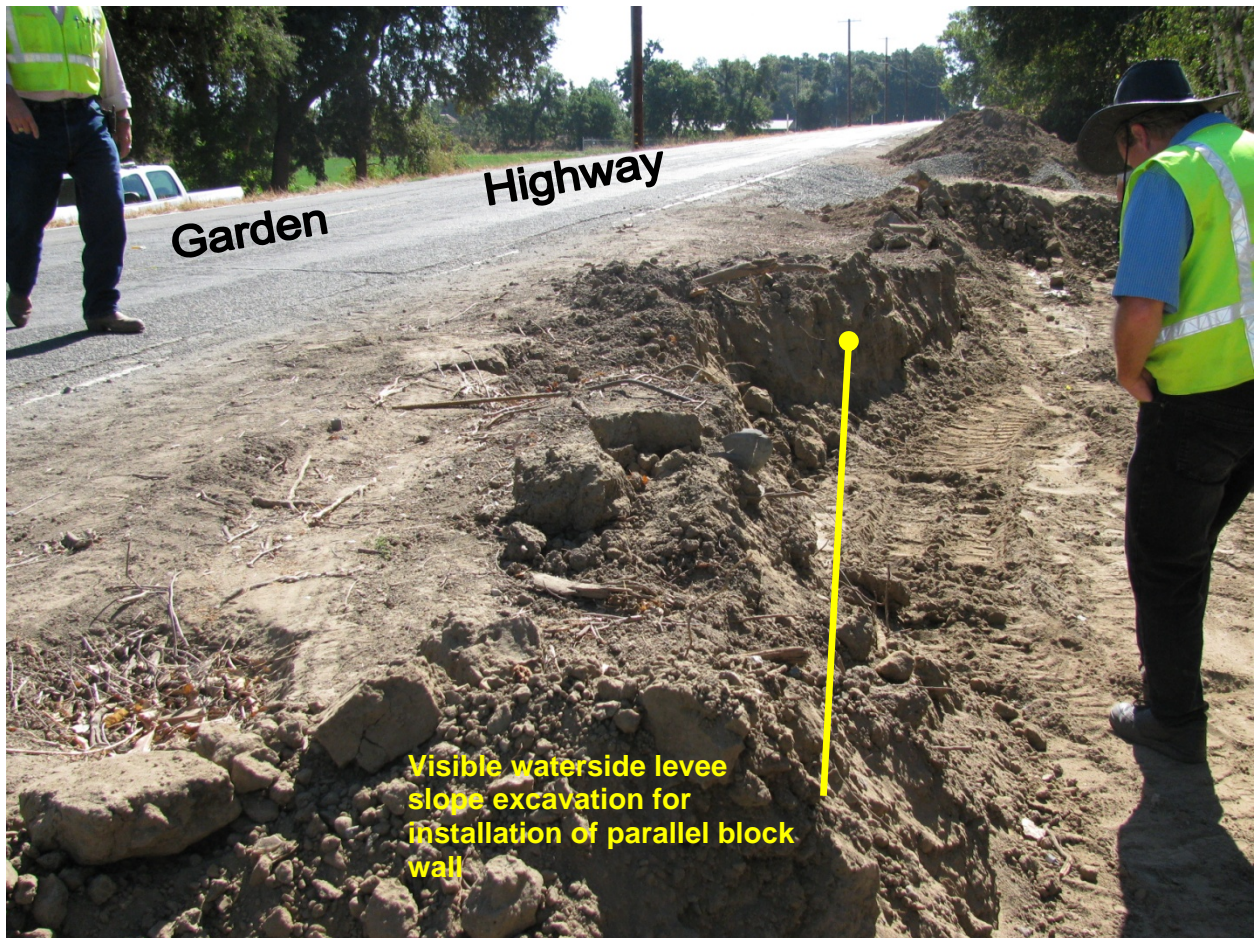
Figure 2b- Cut on waterside levee slope in preparation for block wall. Board staff site visit on September 21, 2010.
