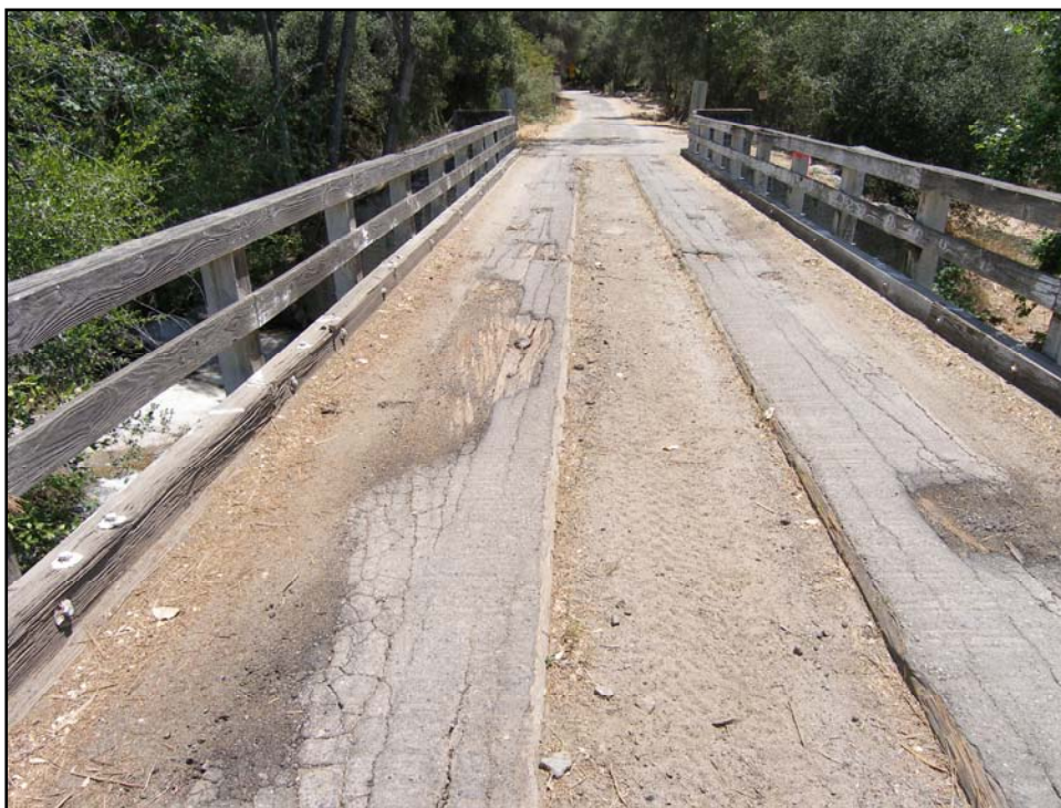
View southeast along Bridge 46 C0119, showing deterioration of roadway surface timbers.
