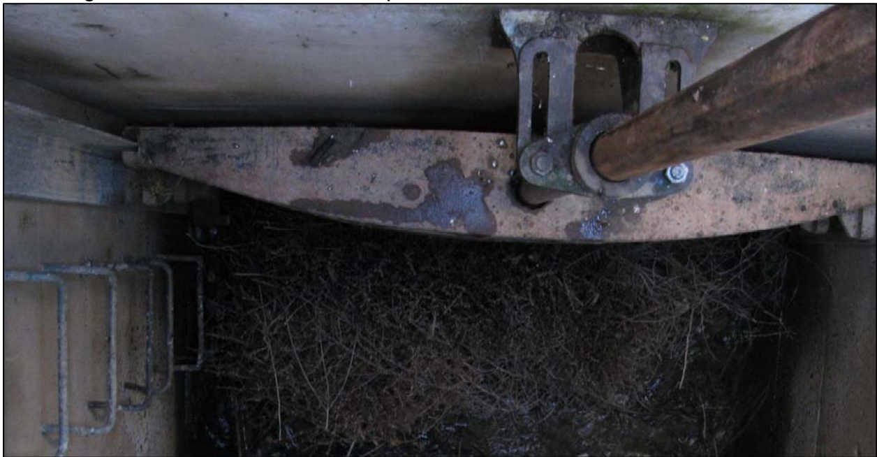
2 – Looking down on the gate at the existing 6'x4' box culvert, notice debris
