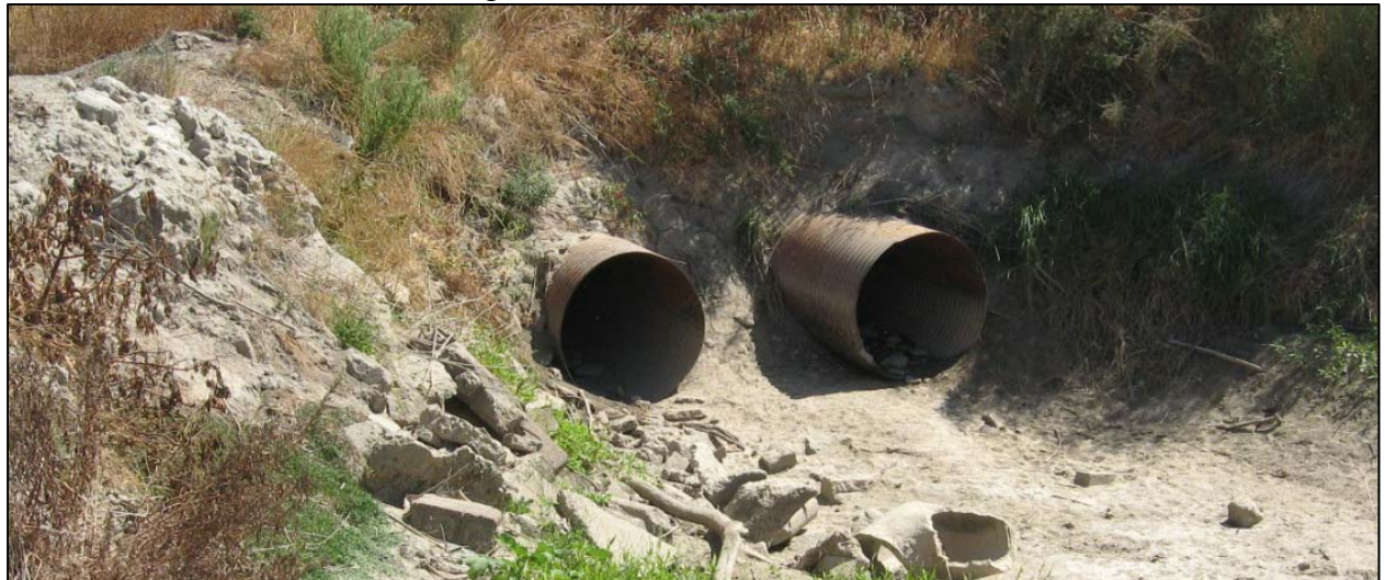
3 – Downstream side of existing two, 48-inch diameter CMP culverts on Sep. 23, 2010.
