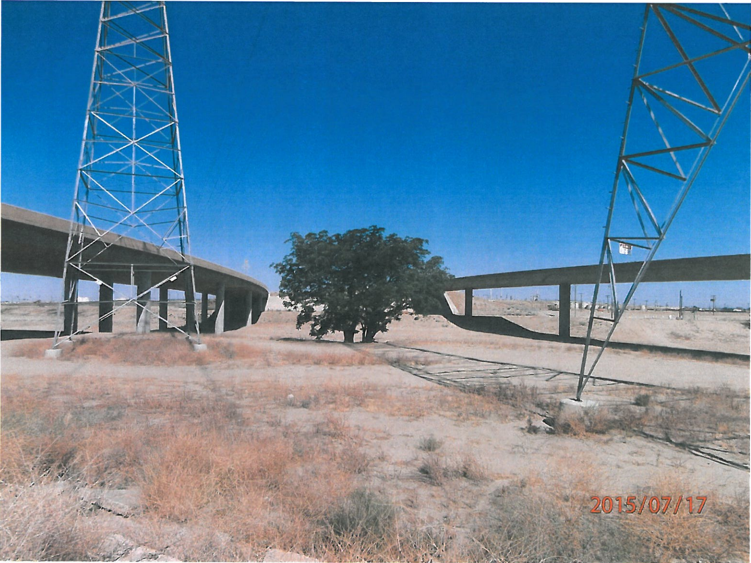
Photo #3 Facing north toward Kern River between Westside Parkway bridges (July 17, 2015)
