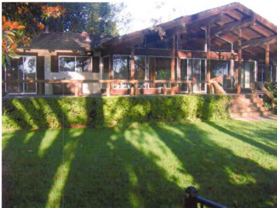
Photo 4. View of the first floor elevation from the front yard
