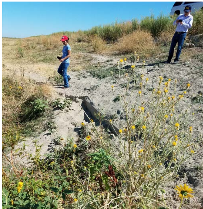
Photo 2: Reach O-1 levee and 24-inch culvert penetration on inside toe of levee, looking downstream. Source: California Department of Water Resources 2018
