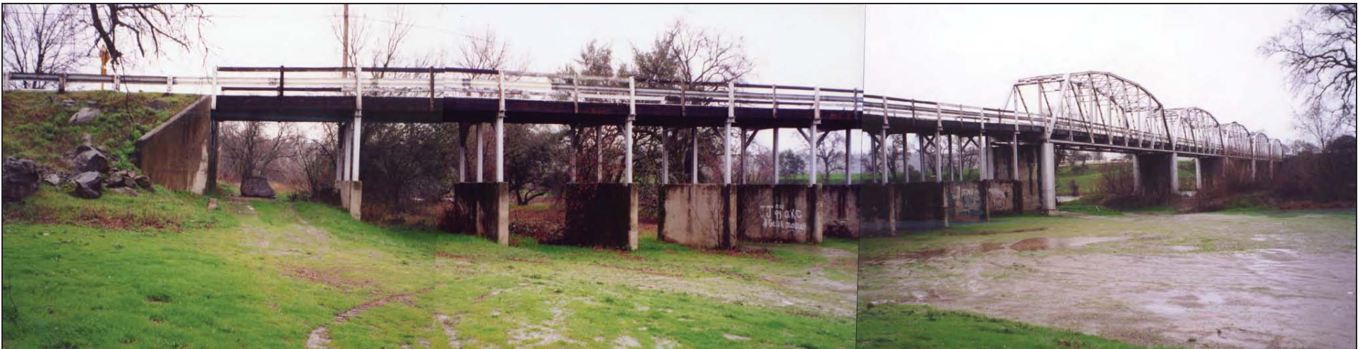
Photo 2: Looking downstream (southeast) at Bridge 8C-0043, Jellys Ferry Road over Sacramento River
