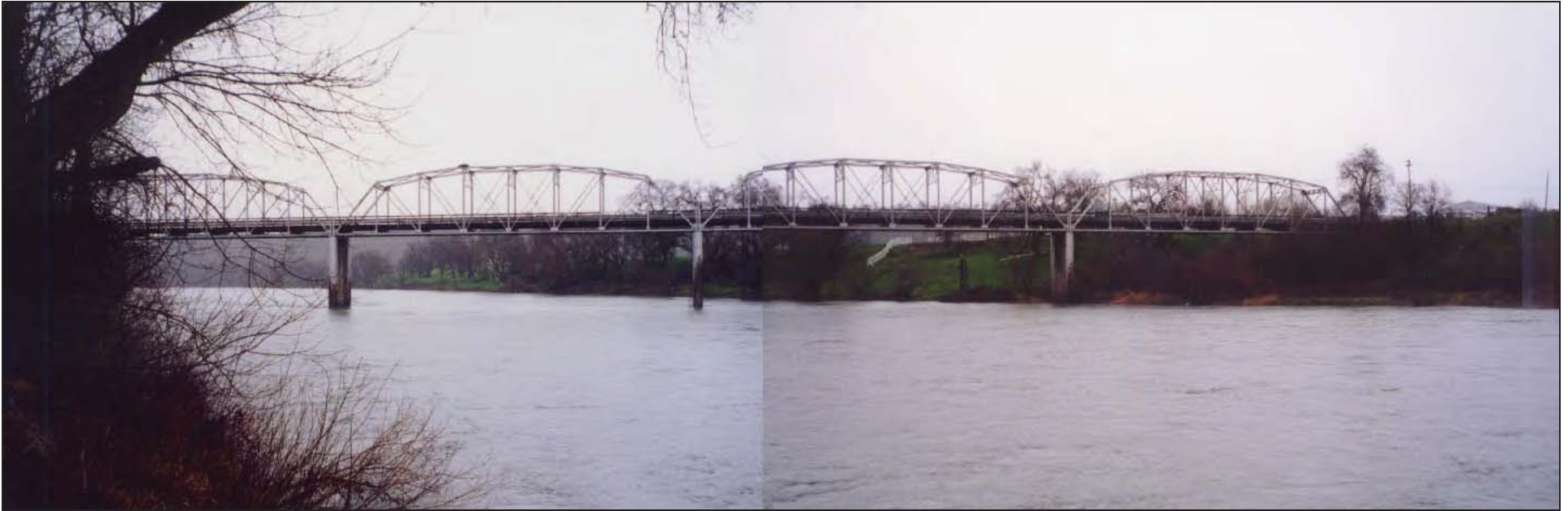
Photo 1: Looking downstream (east) at Bridge 8C-0043, Jellys Ferry Road Bridge over Sacramento River
