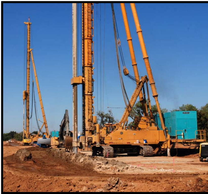
Figure 6. Slurry (Cutoff) Wall Construction Using DMM.
