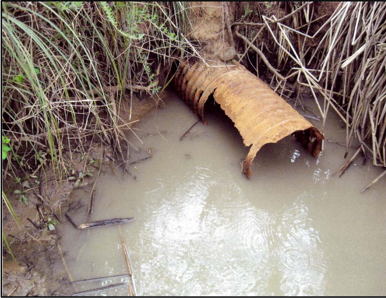
Figure 3. WPIC damaged culvert to be replaced
