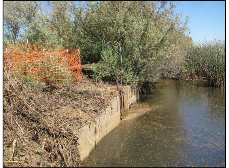
Figure 4. WPIC headwall to be replaced
