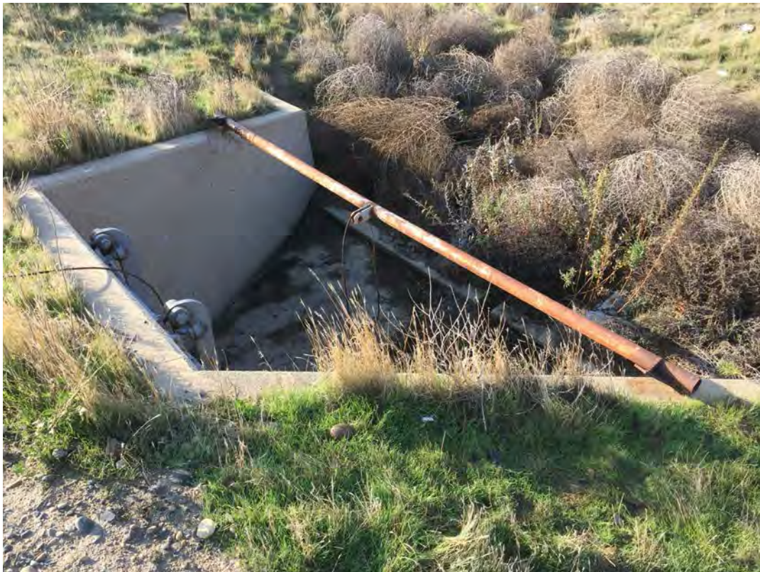
Figure 4. View of existing box culvert, flap gate, and wing wall on waterside levee toe
