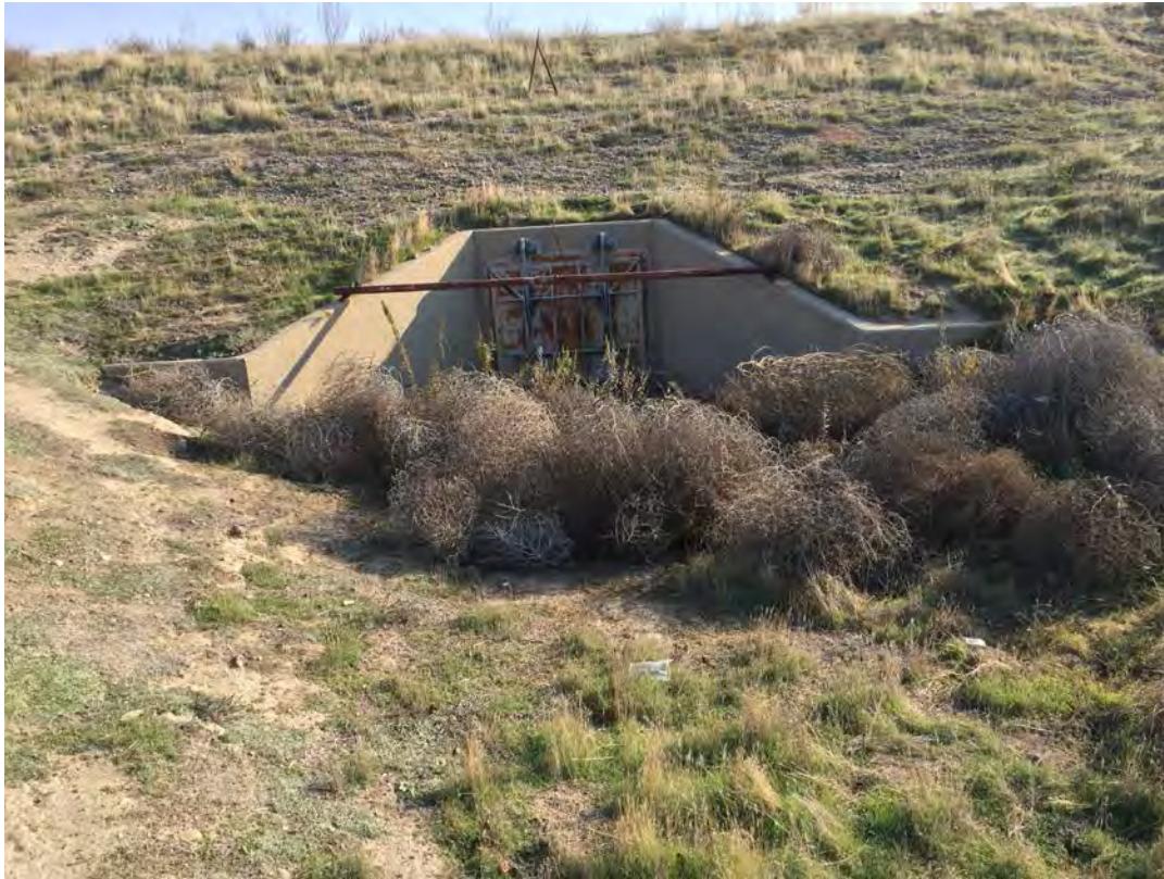
Figure 3. View of existing box culvert, flap gate, and wing wall on waterside levee toe
