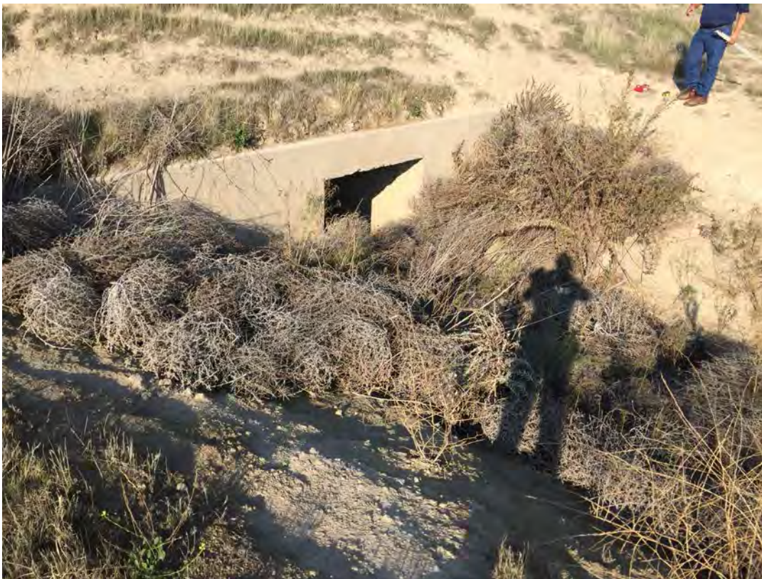
Figure 6. View of existing box culvert and wing wall on the landside levee toe
