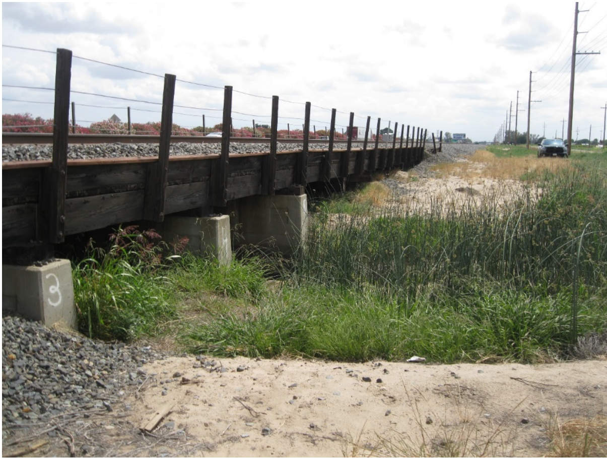
Photograph 2. View to the southwest within the western ROW.
