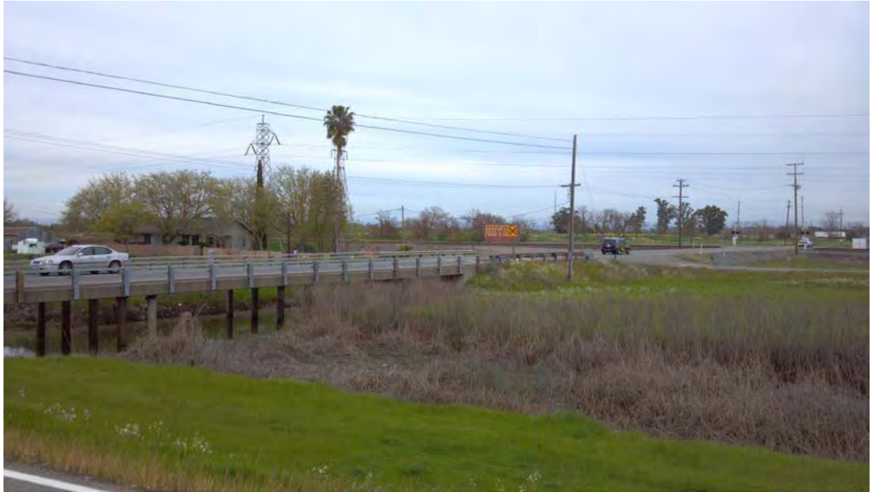
East Natomas Main Drain - Looking Northeast 3/18/2013
