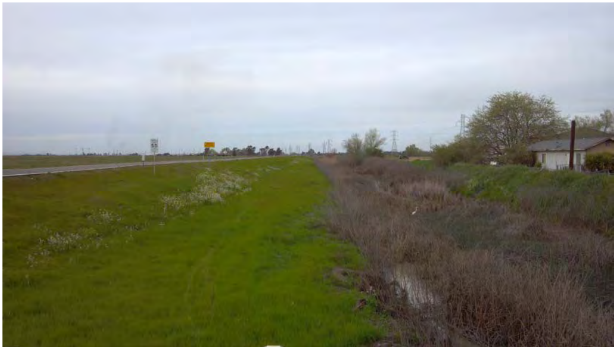
East Natomas Main Drain - Looking North 3/18/2013
