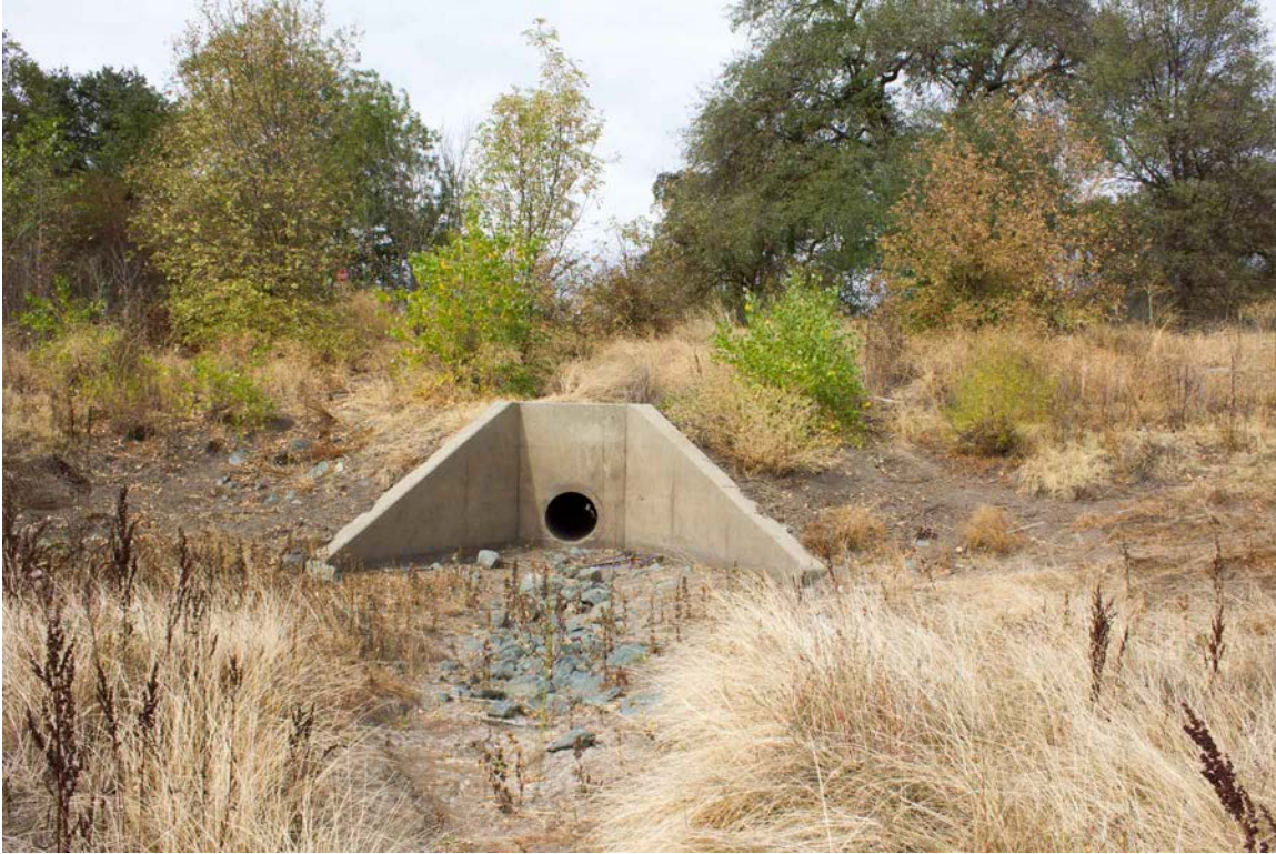
Photo 1. View looking north from within the basin towards the existing 30" culvert. The invert can be seen to be higher than some of its surroundings, forming fish entrapment pools when the basin has partially filled and then receded.
