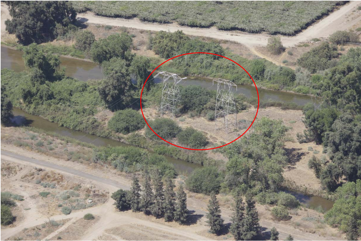
High voltage towers inside the St. John's River Floodway.
