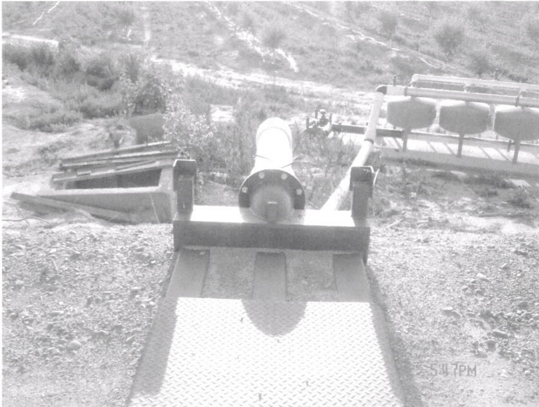
View to upland from levee crown of temporary pipe configuration
