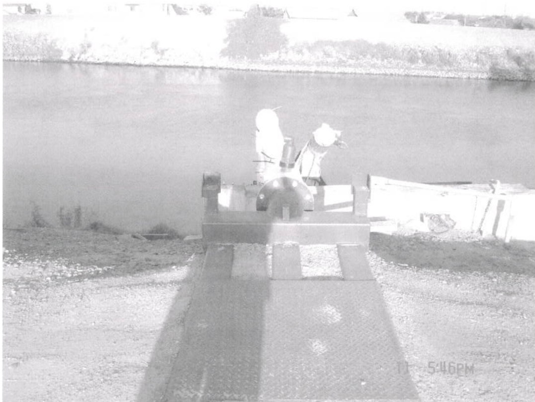
View across river from levee crown of temporary pipe configuration
