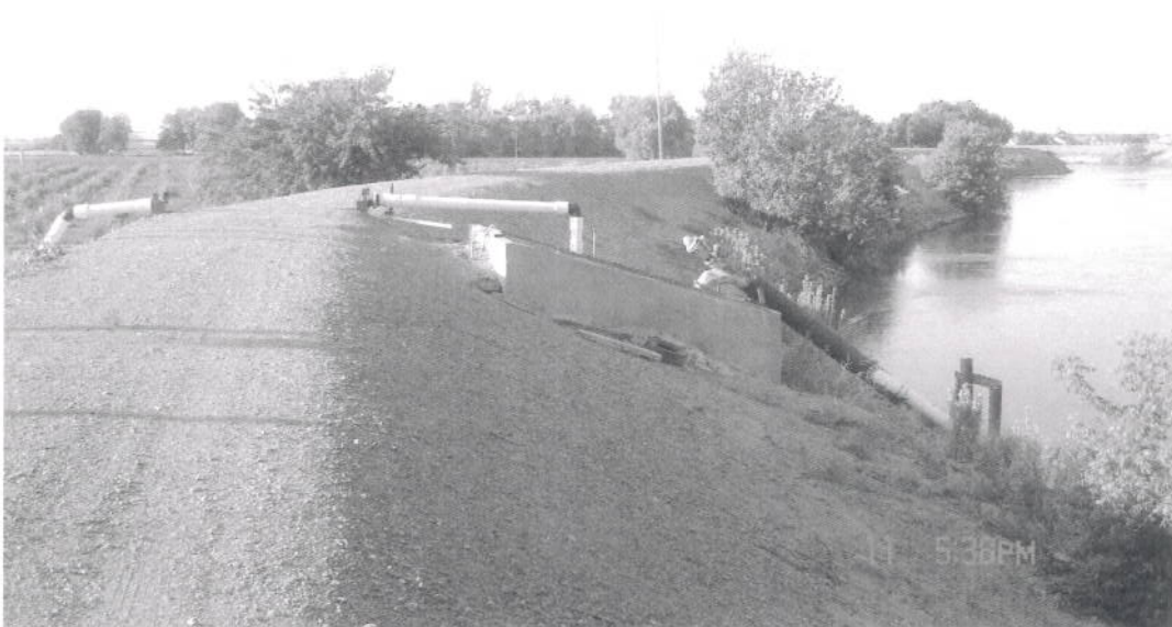
Upstream view of temporary pipe configuration and existing pipe
