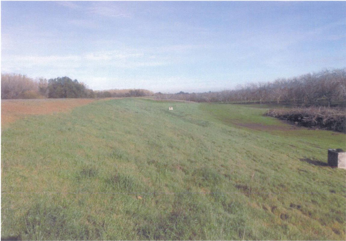
B. Feather East Levee Landside Station 133+00 – Looking North December 2012
