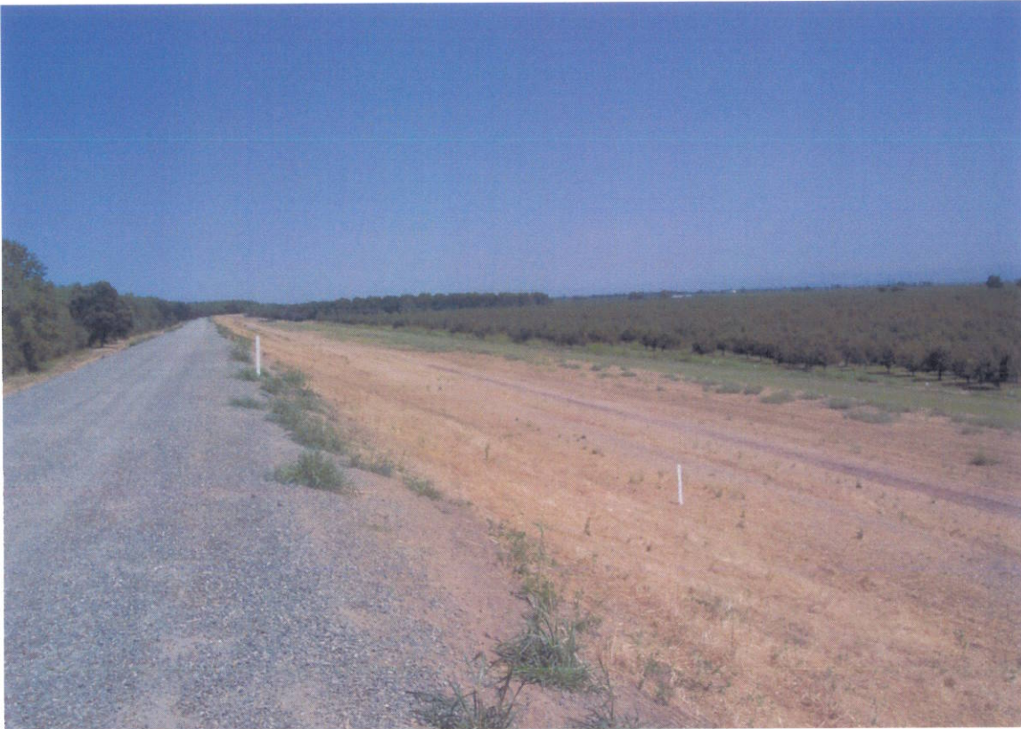
D. Feather East Levee Landside Station 100+00 – Looking North August 2010
