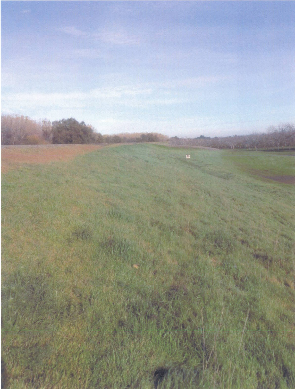
A. Feather East Levee Landside Station 133+00 – Looking North December 2012
