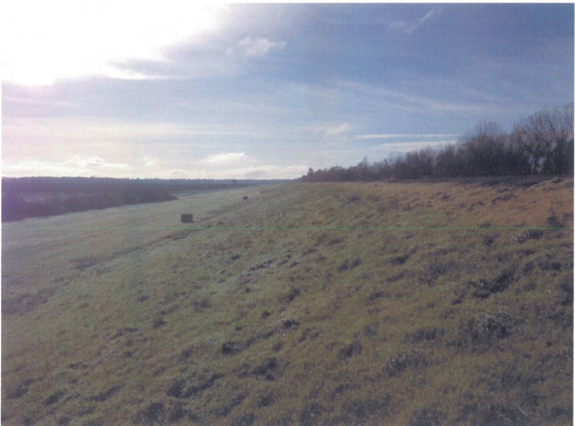
C. Feather East Levee Landside Station 133+00 – Looking South December 2012
