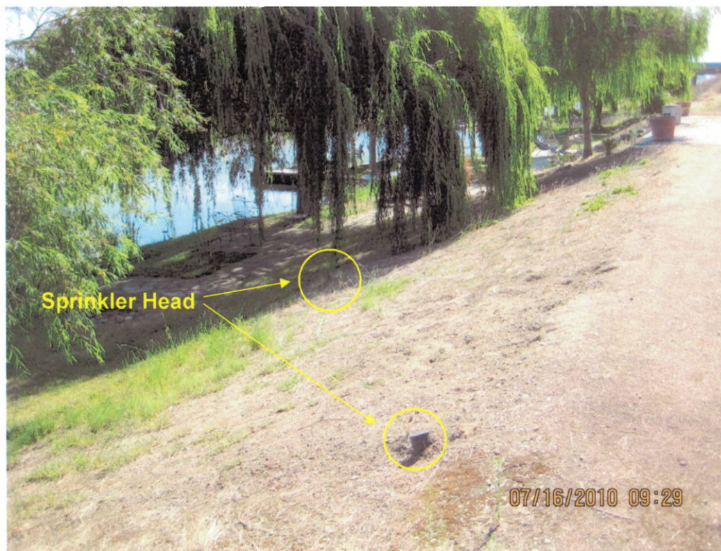
Figure 3 Sprinkler system at the levee waterside; the red apple ice plant has been removed.
