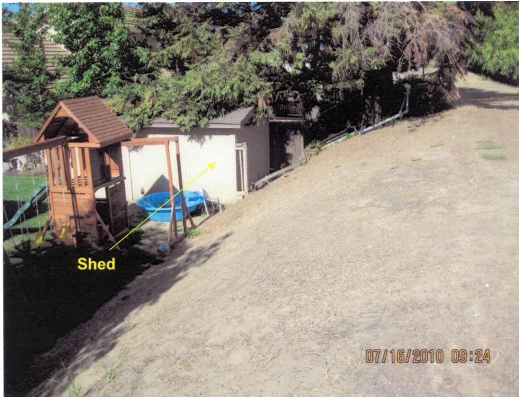
Figure 2 Wood shed at the western edge of property (levee landside); most of the encroachments have been removed.
