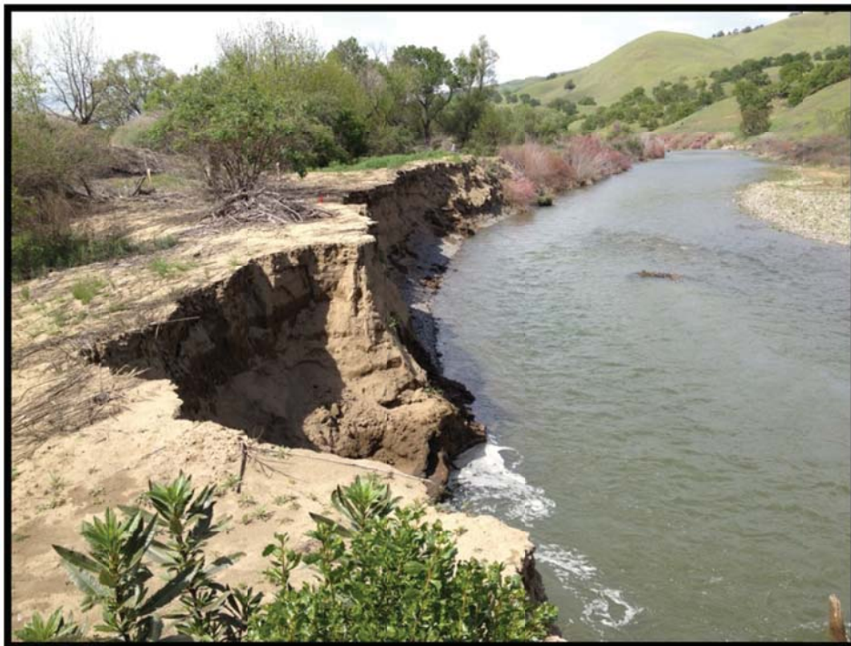
Photo 2: Upstream view of eroding bank taken from southern point of proposed Longitudinal Stone Toe Protection. (Photo taken April 16, 2012).
