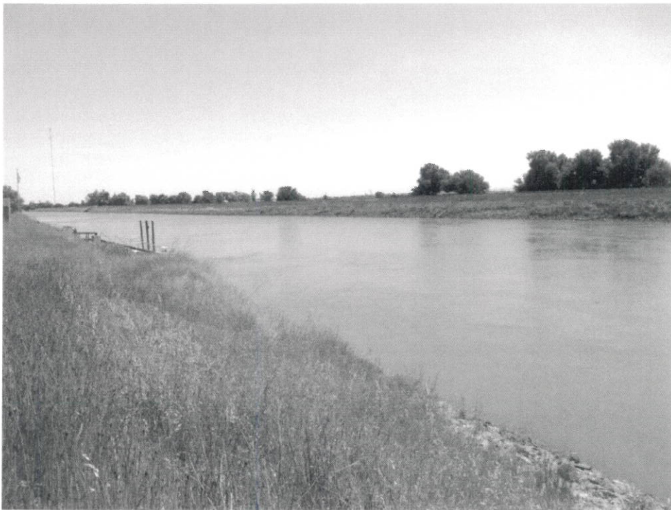
Downstream view from project site.
