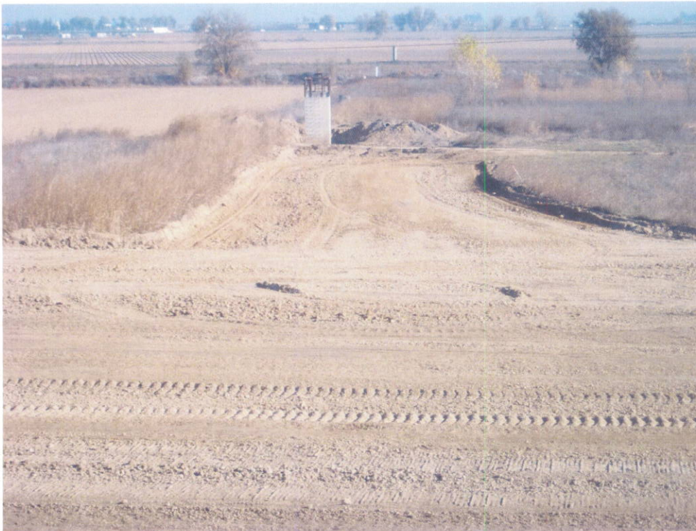
Photograph 4: Looking east from top of new adjacent levee at Siddiqui River Pump.
