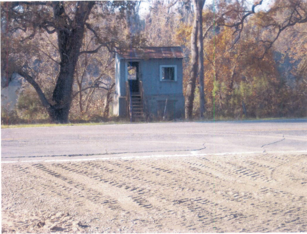
Photograph 3: Looking west from top of new adjacent levee at Siddiqui River Pump.
