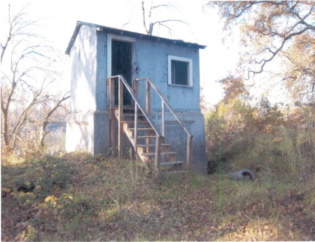
Photograph 1: Siddiqui River Pump existing pump house (River Mile 69.15)
