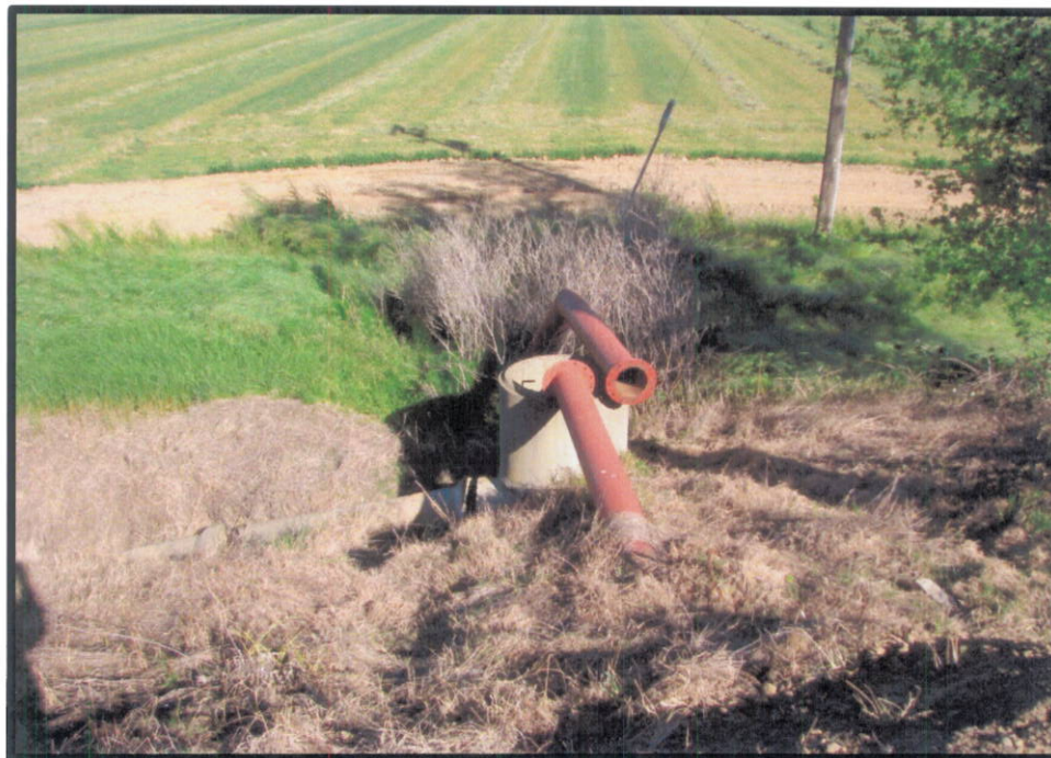
View of landside slope and concrete to be removed.
