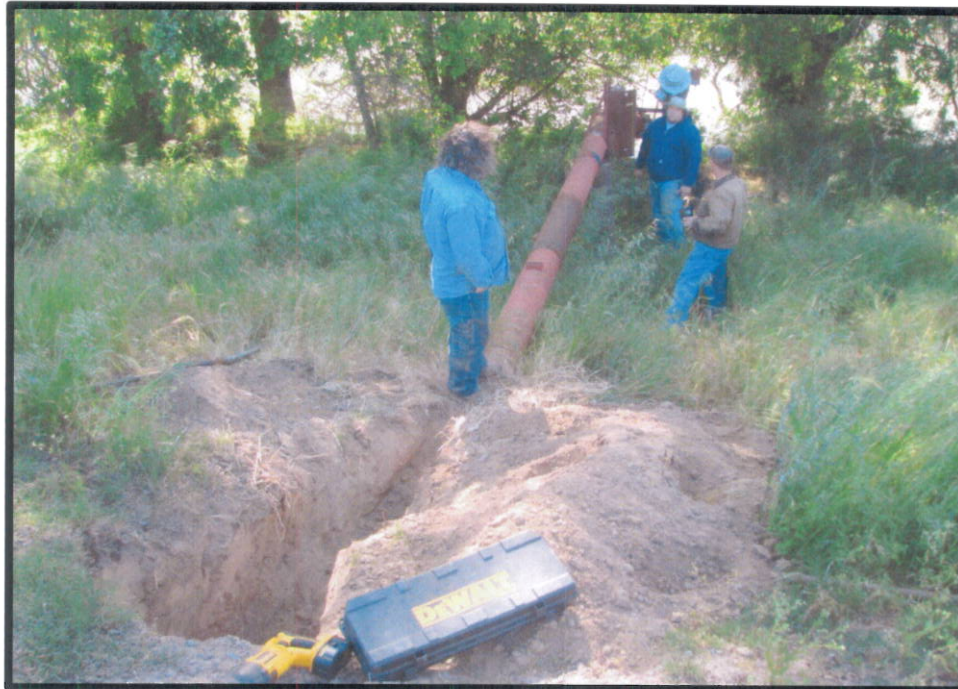
Waterside slope and bank with encroachment under maintenance.
