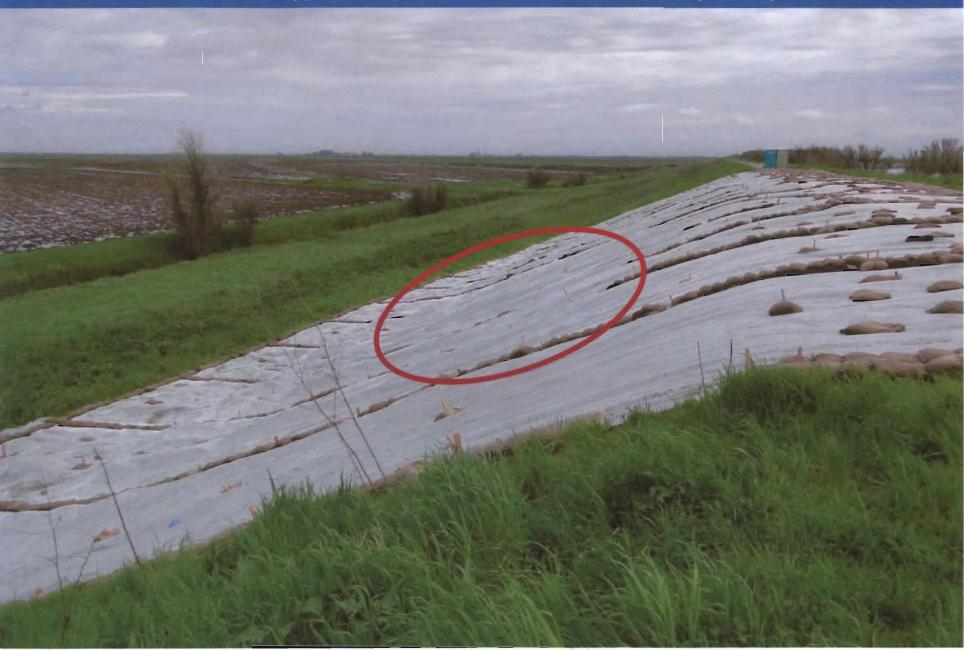
Landside Slope Cracking/Slumping on North Levee of Natomas Cross Canal (RD 1001) View Looking West (03-27-11)
