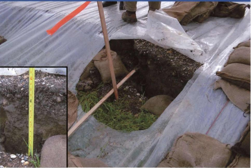
Landside Slope Cracking/Slumping on North Levee of Natomas Cross Canal (RD 1001) View of Apparent Bulging on Lower Slope - Looking East (03-27-11)
