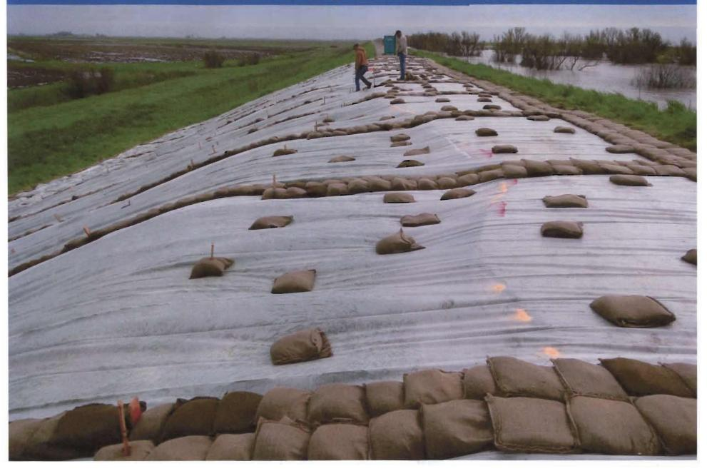
Landside Slope Cracking/Slumping on North Levee of Natomas Cross Canal (RD 1001) View of Upper Slide Scarp Through Cut in Plastic (03-27-11)
