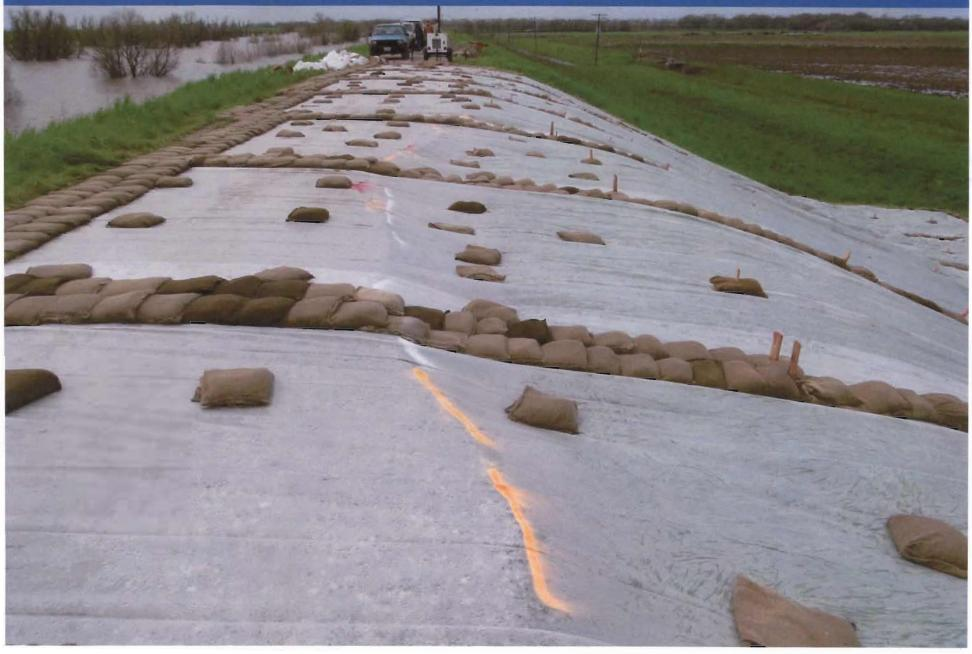
Landside Slope Cracking/Slumping on North Levee of Natomas Cross Canal (RD 1001) Progression of Eastern Edge of Cracking on Levee Crown - March 26 and March 27 - Looking West (03-27-11)
