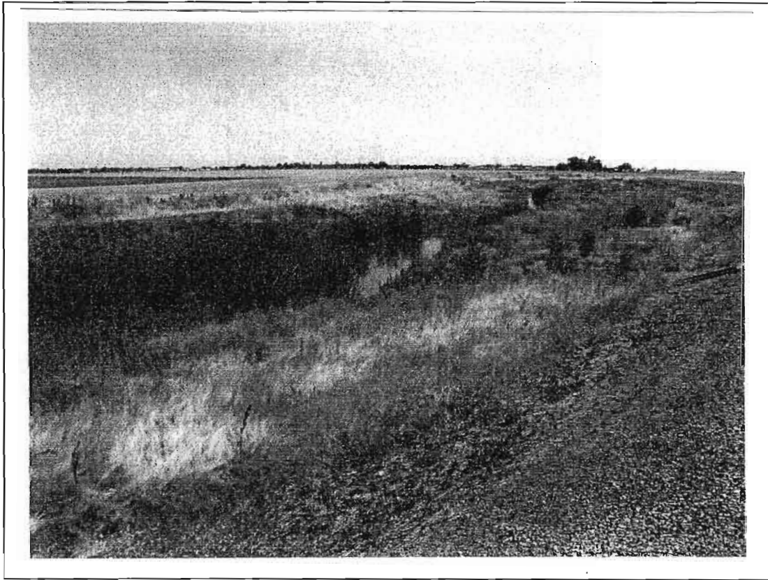
Approximate location of the proposed outfall structure at the southern edge of Bear Creek, looking east; 6/13/03
