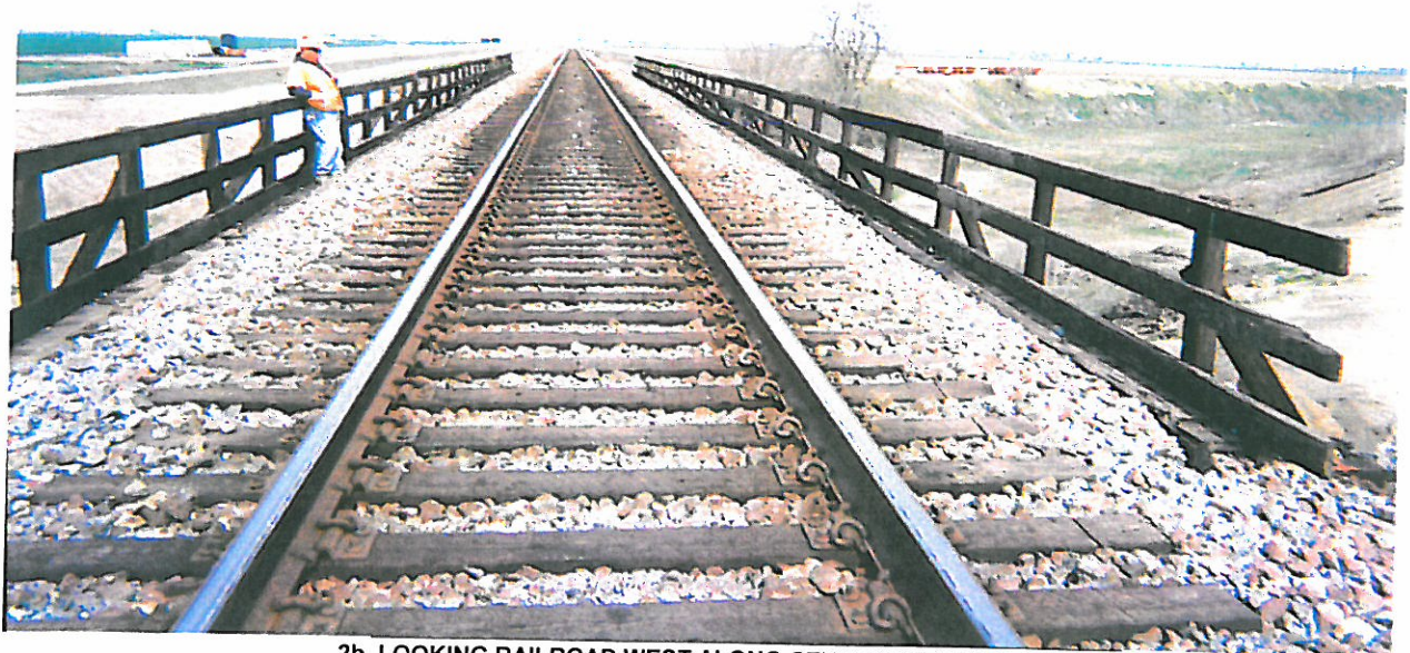
2b. LOOKING RAILROAD WEST ALONG CENTERLINE OF TRACK
