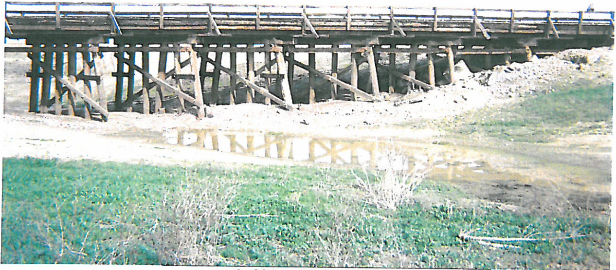
6a. SOUTH FACE OF BRIDGE
