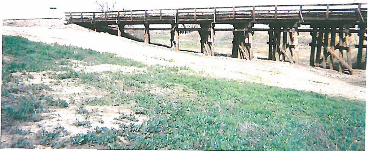
6b. SOUTH FACE OF BRIDGE
