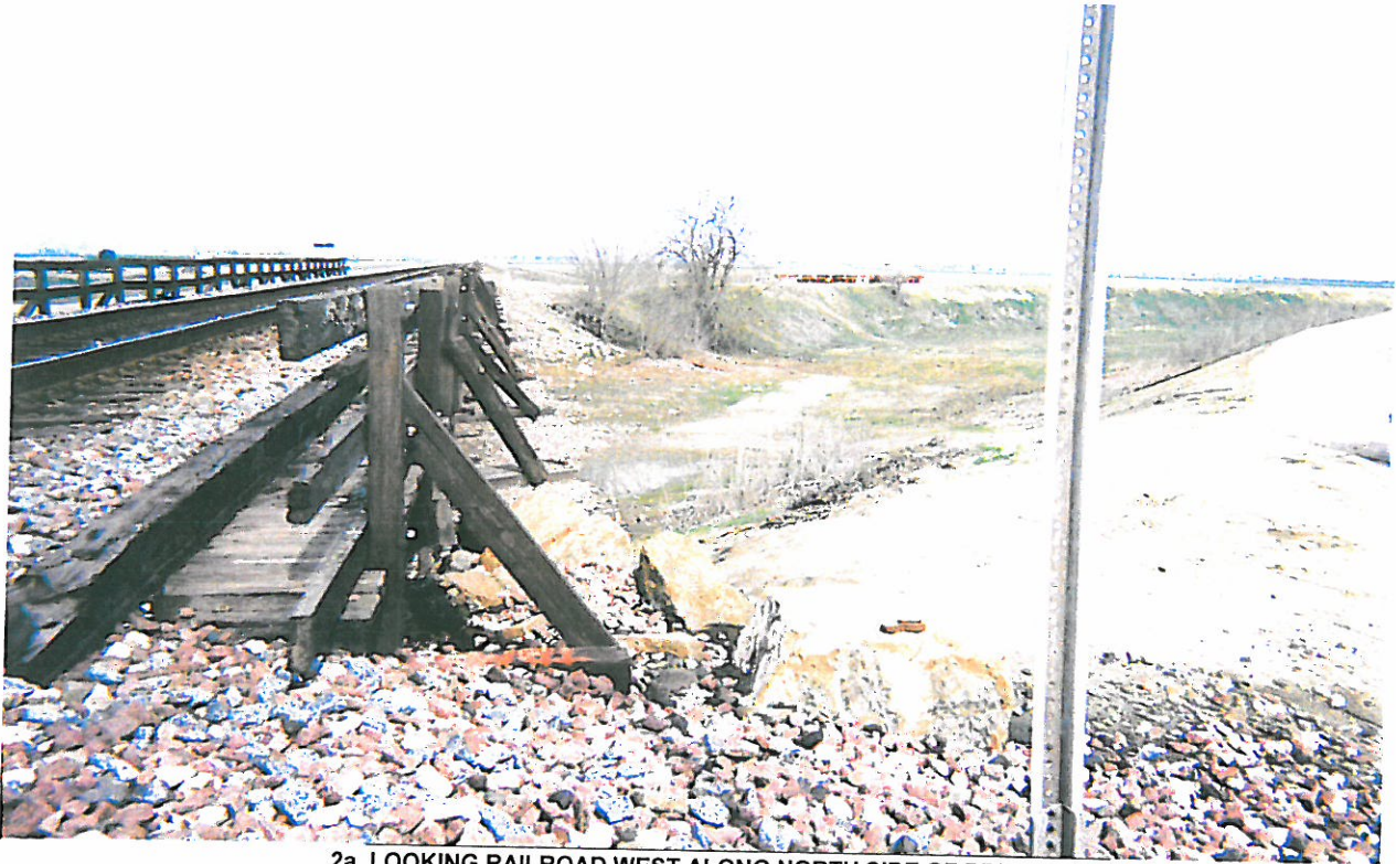
2a. LOOKING RAILROAD WEST ALONG NORTH SIDE OF BRIDGE
