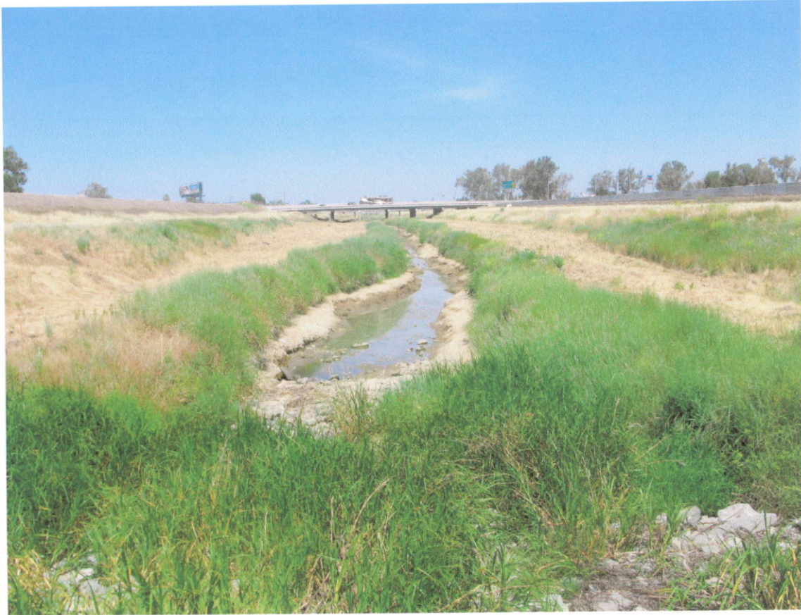
Figure 3. Photo depicting current conditions, looking downstream from flashboard dam
