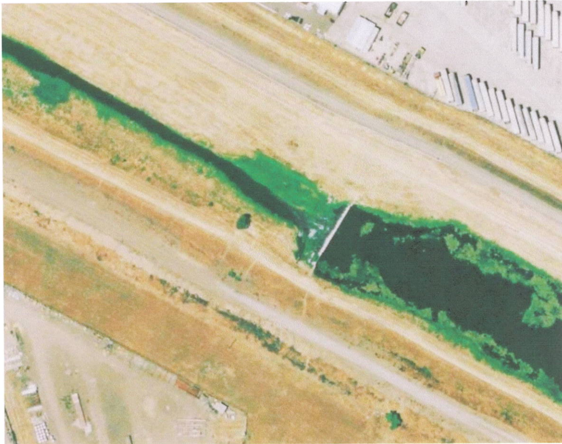
Figure 1. Aerial photo of Budiselich Dam depicting current conditions with flashboards installed. The rock weir structures will be downstream of the flashboard dam (top left).
