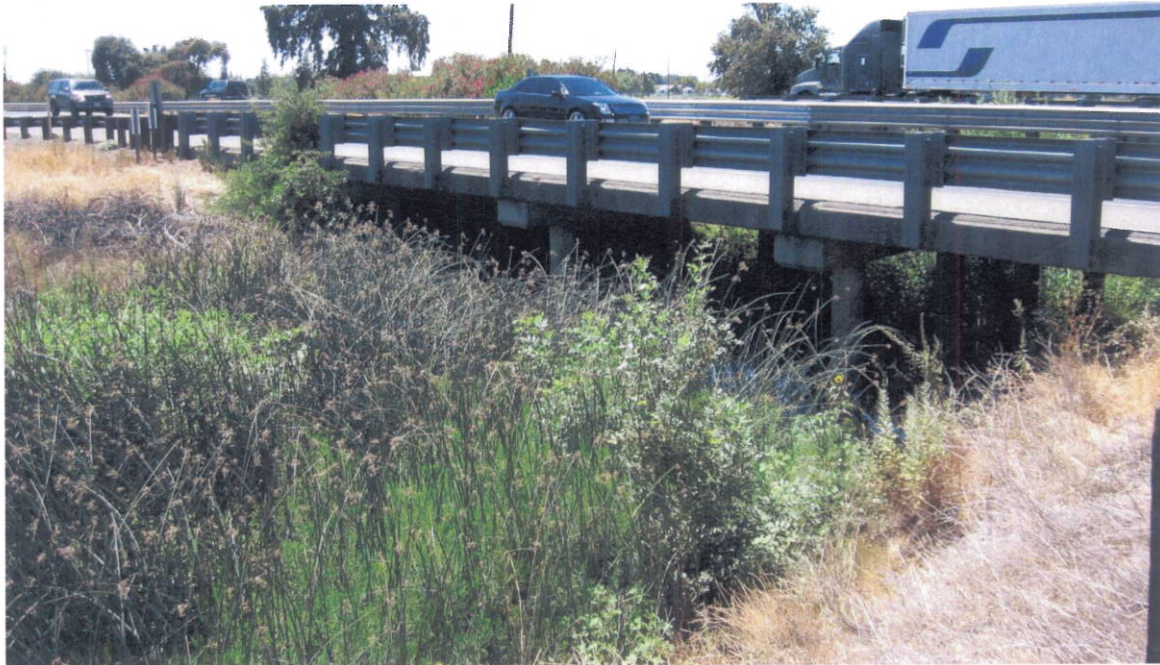
Figure 7. View of bridge looking southwest.
