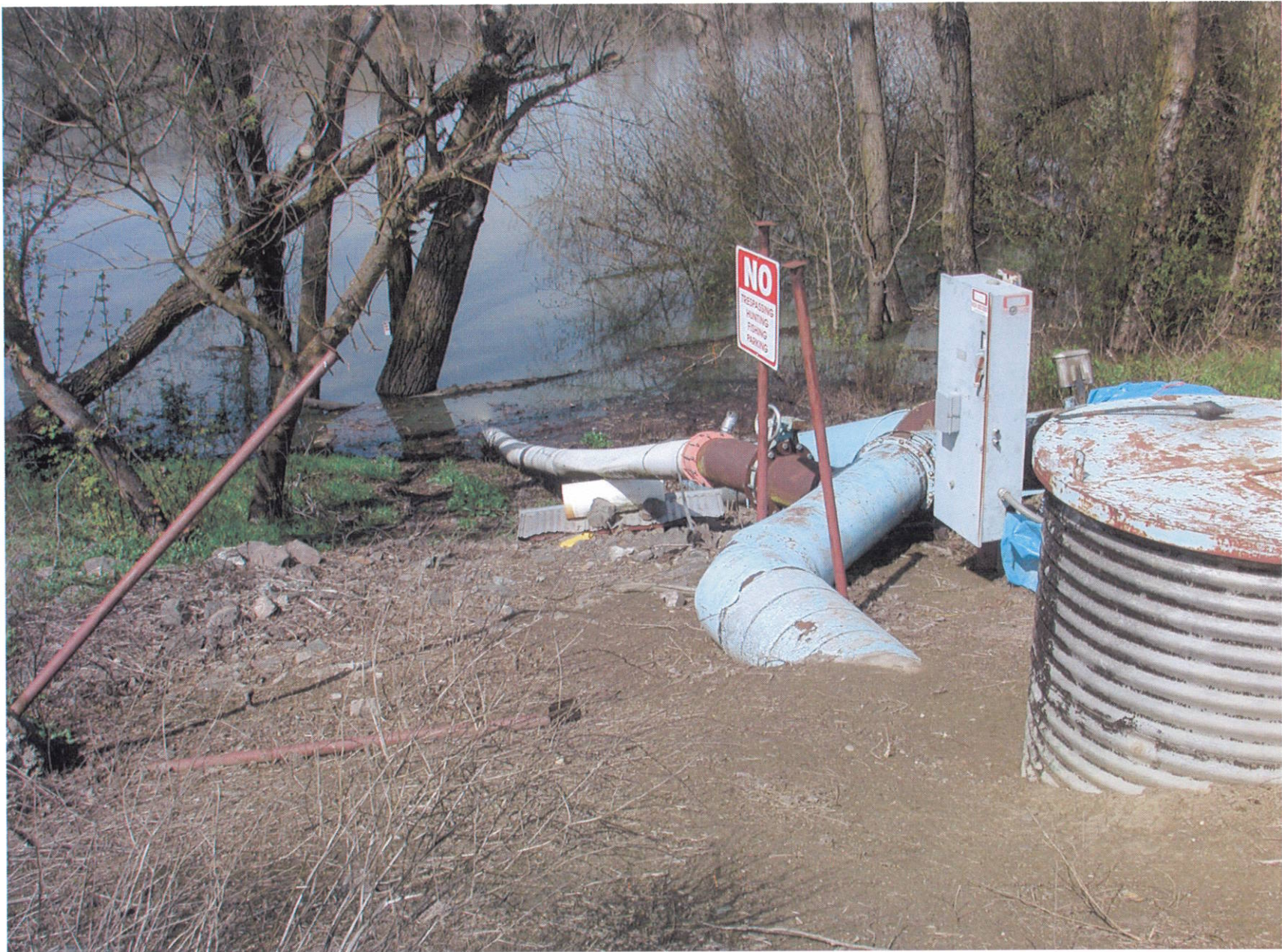
LOOKING WEST TOWARDS THE RIVER FROM THE TOP OF THE LEVEE
