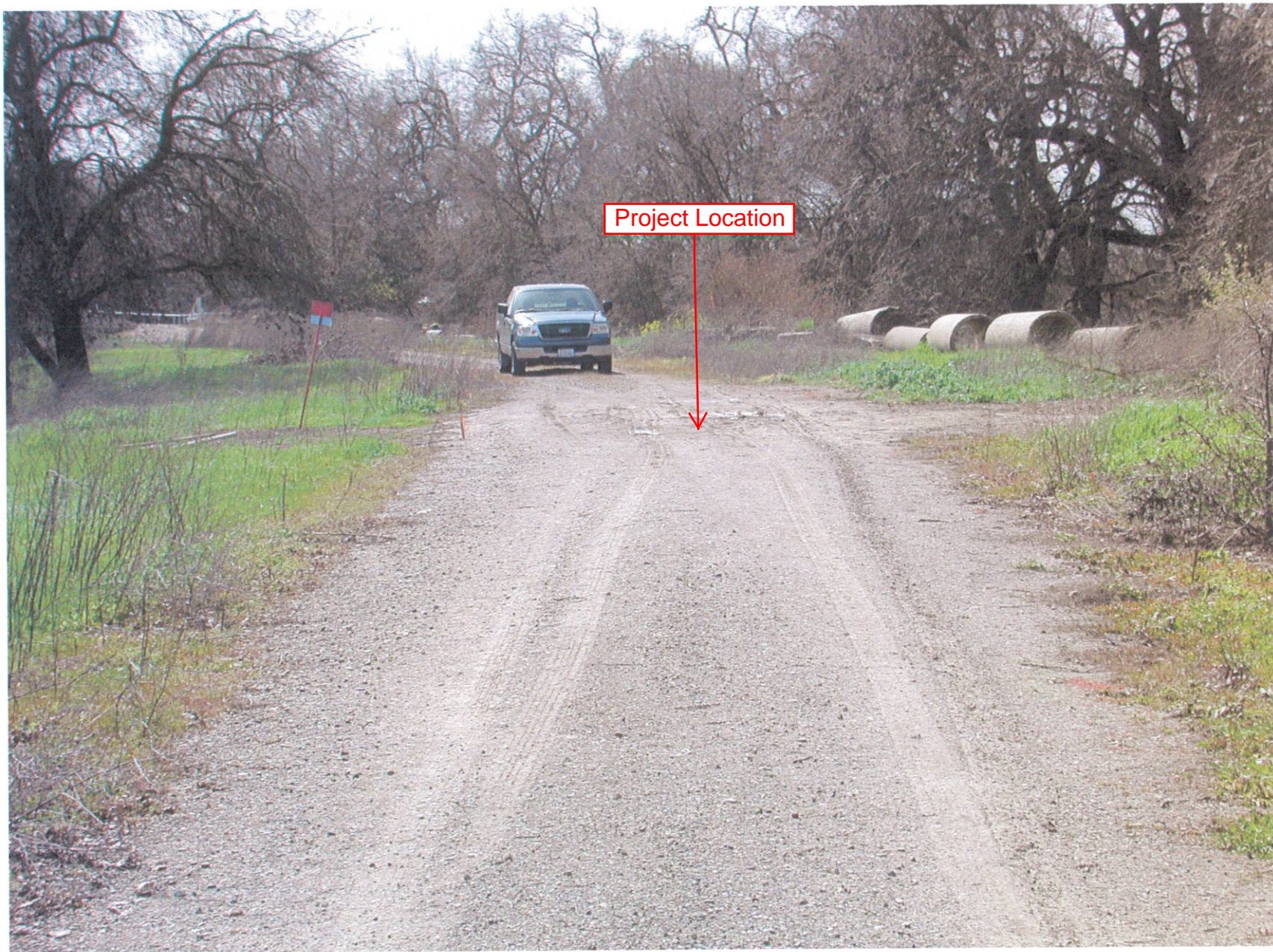
LOOKING SOUTH FROM THE TOP OF THE LEVEE
