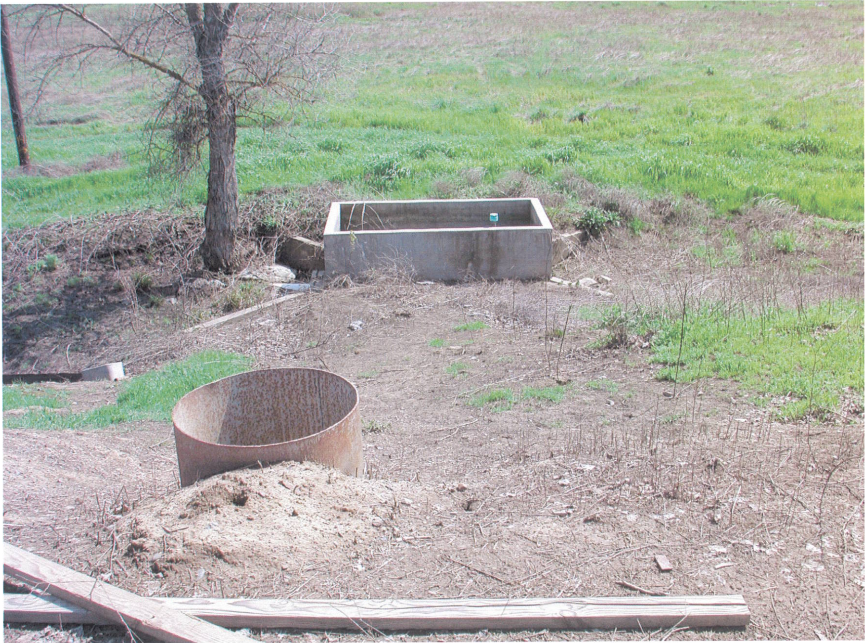
LOOKING EAST (LAND SIDE) FROM THE TOP OF THE LEVEE
