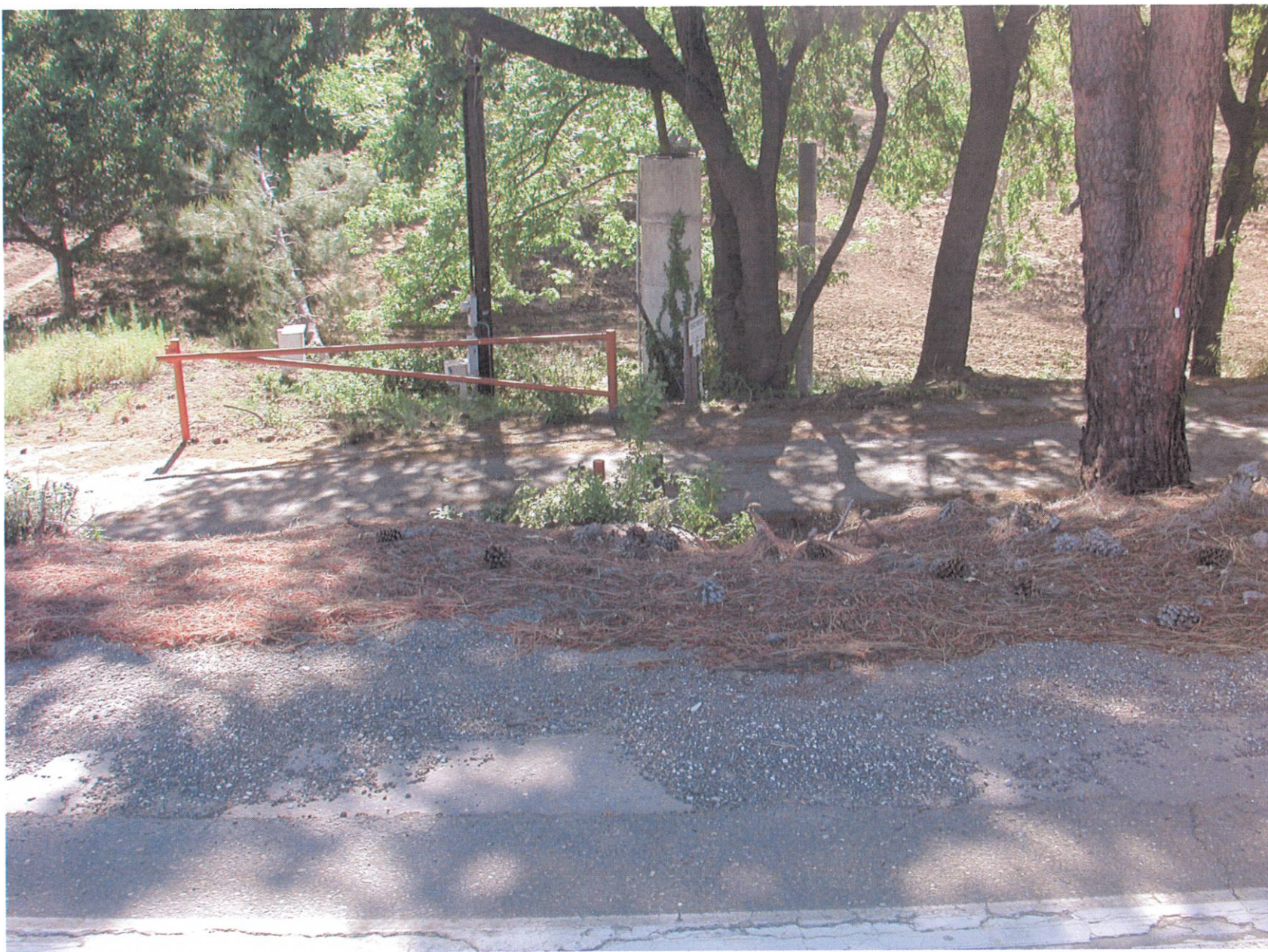
LOOKING TOWARDS LAND SIDE FROM TOP OF LEVEE
