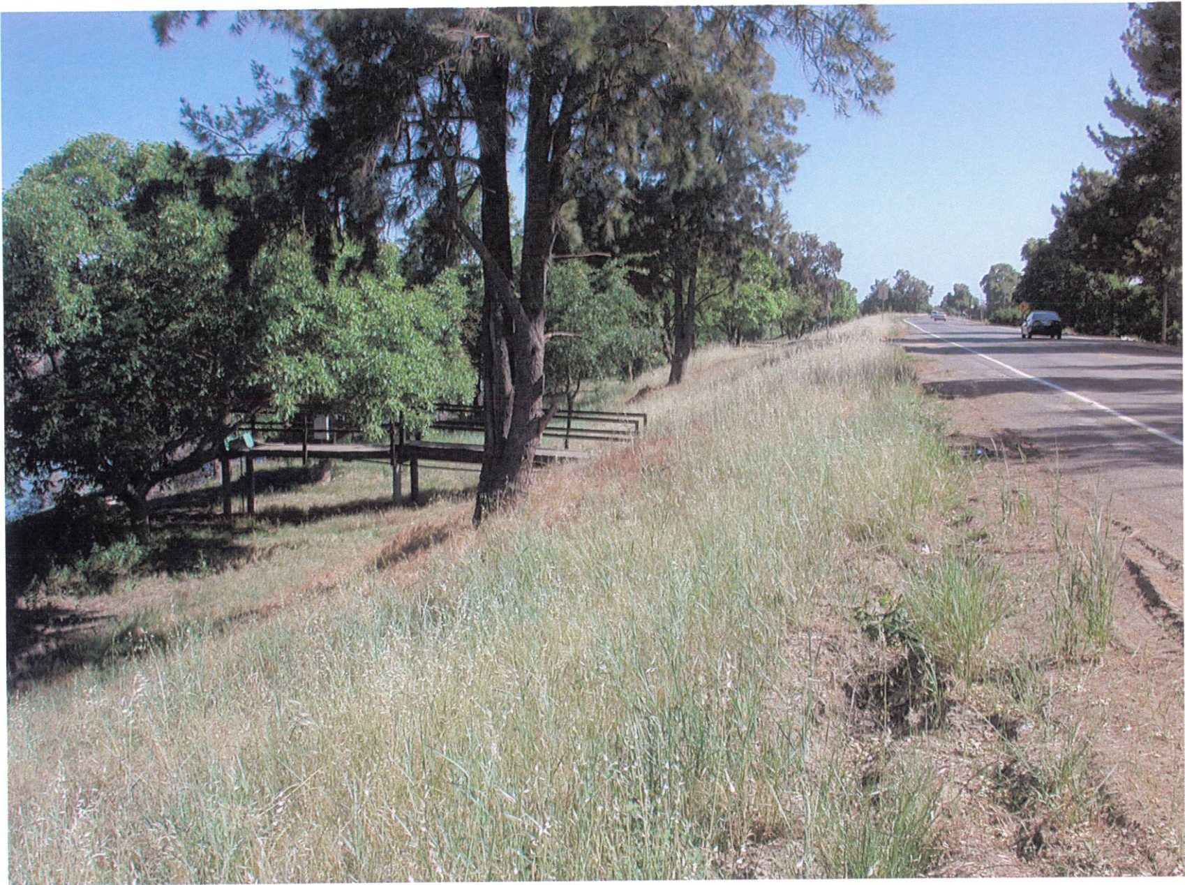
LOOKING SOUTH FROM TOP OF LEVEE
