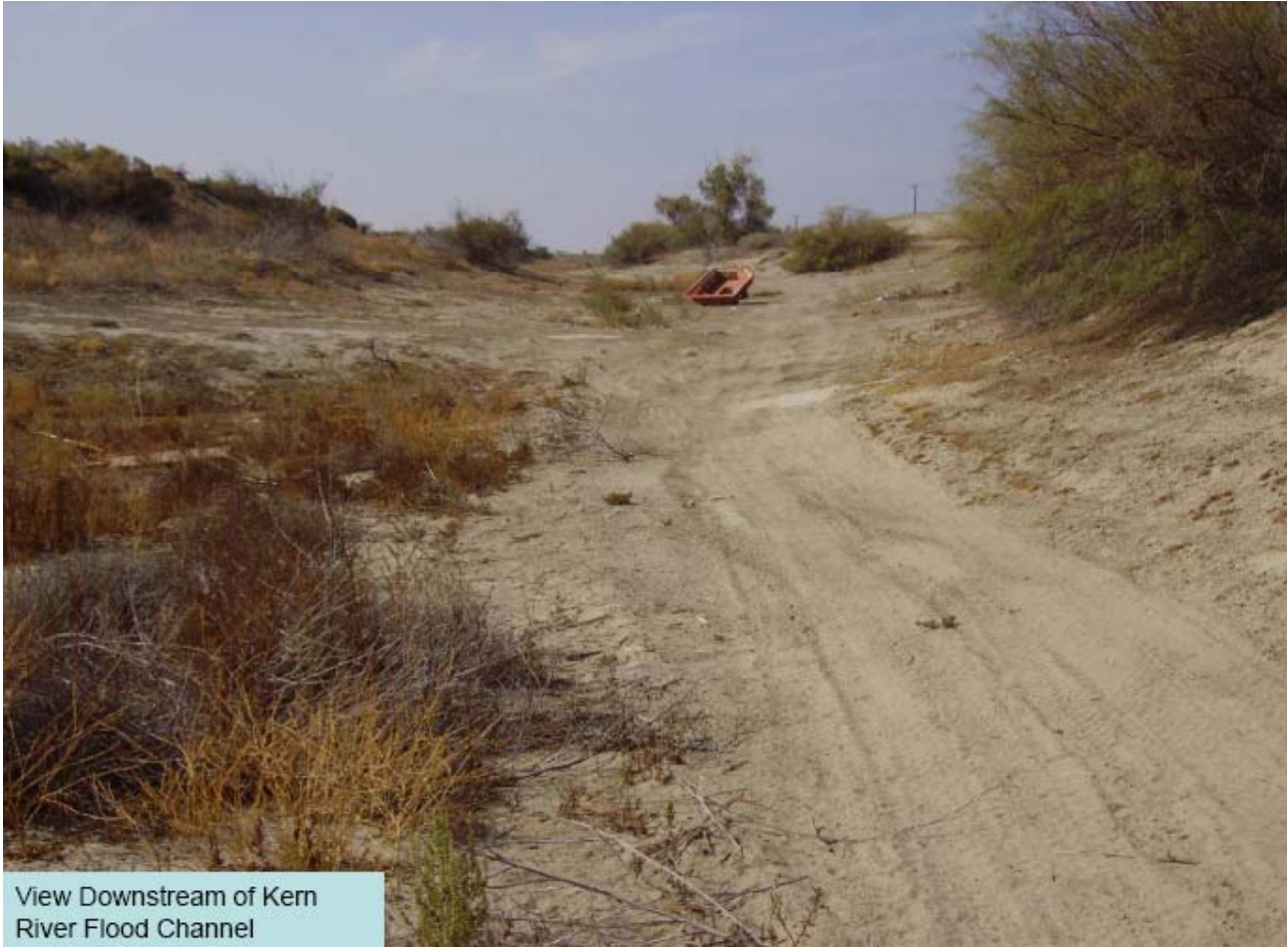
View Downstream of Kern River Flood Channel from NE Bank
