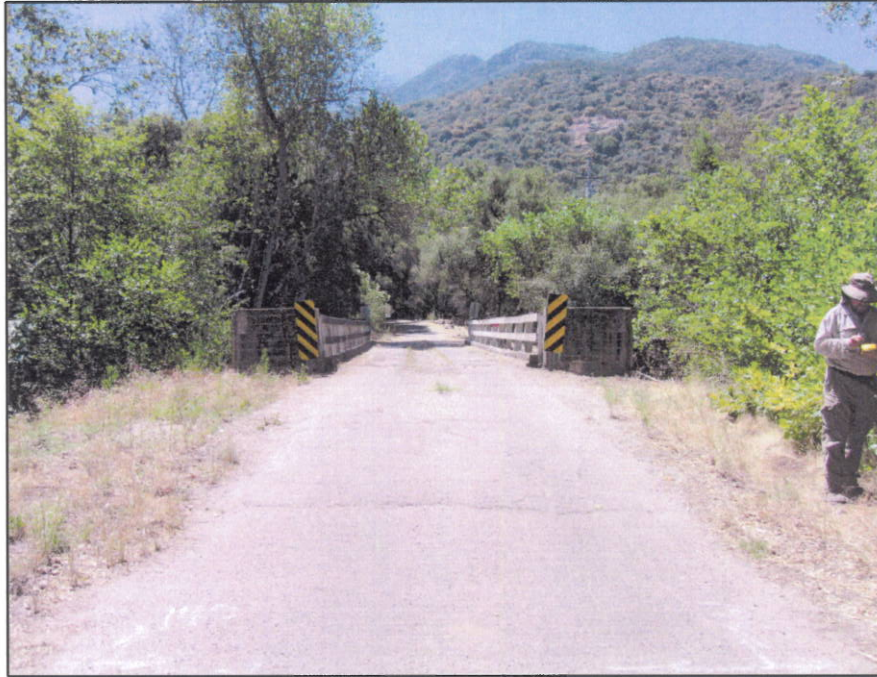
Photo 1: Northern approach to existing bridge
