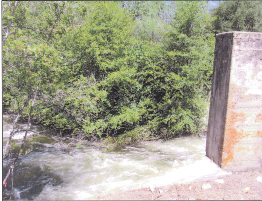
Photo 3: Downstream view from north end of existing bridge
